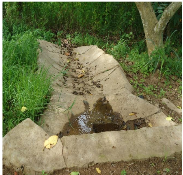
Overflow point on Northern side of the existing road
