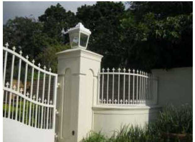
Exterior view of the gates/feature walls
