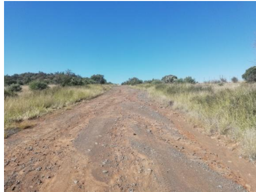
Existing access road to the property and site.
