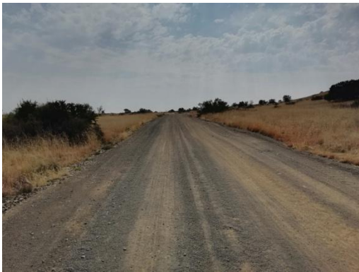
Existing gravel access road to the proposed project site.
