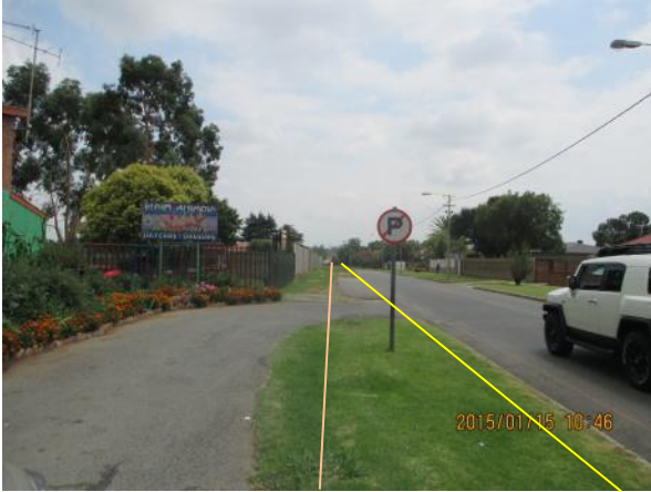
Photo 5: After crossing Ermelo Road the pipeline is routed on the pavement along Lake Road.
