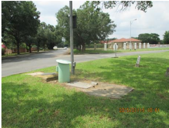
Photo 1: Connection point of the pipeline.
