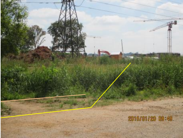
Photo 28: Area where the pipeline route turns left and cross the storm water channel and railway line as it moves toward the AMD treatment plant
