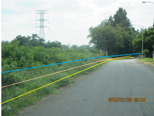
Photo 20: The route along Dyer Road. An unlined, storm water channel runs parallel to the route and Dyer Road (the pipeline route (blue line) is located between the channel and road.
