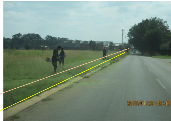
Photo 17: The route along Partridge Road.
