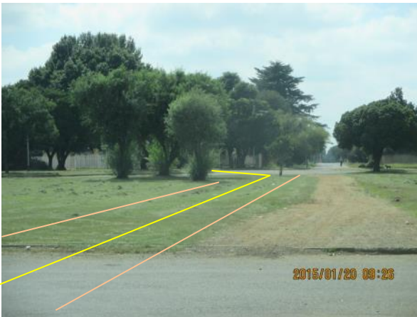
Photo 11: The route crosses Mc Comb Road and a small urban park.
