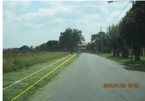
Photo 15: The route along Partridge Road.
