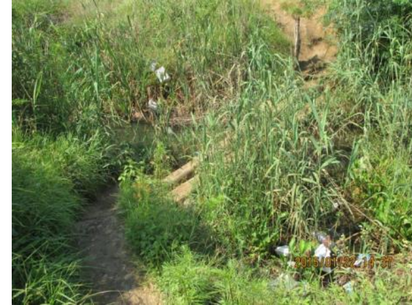
Photo 30: An existing pipe crosses the storm water channel 5 – 10 m upstream of the proposed potable water pipeline crossing.
