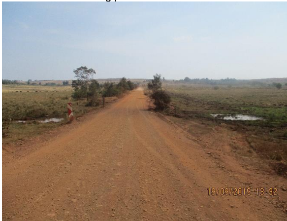
Photo 5: View of the unchanneled valley bottom wetland crossing point at Km 15.520.
