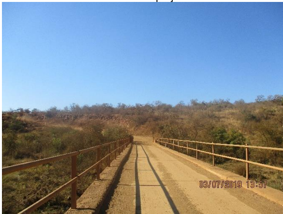
Photo 3: View of the existing single lane bridge over the Mozana River crossing point.
