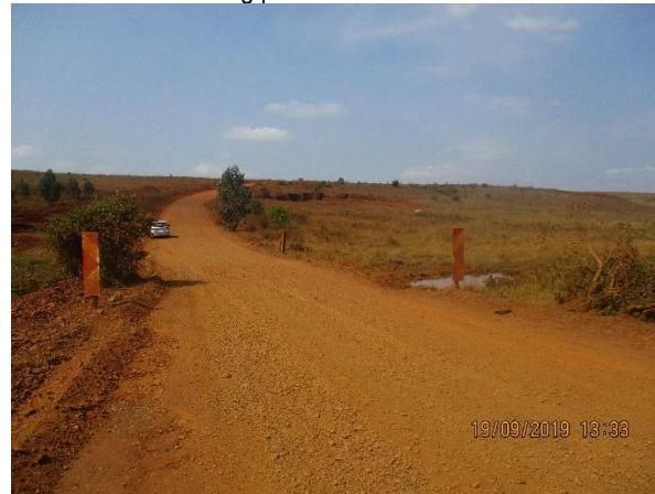
Photo 6: View of the unchanneled valley bottom wetland crossing point at Km 15.520.
