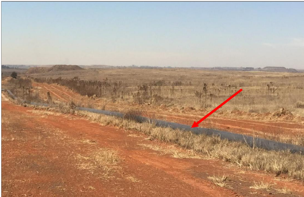
Figure 18: Photograph of existing pipelines (similar pipeline expected for dewatering line)
