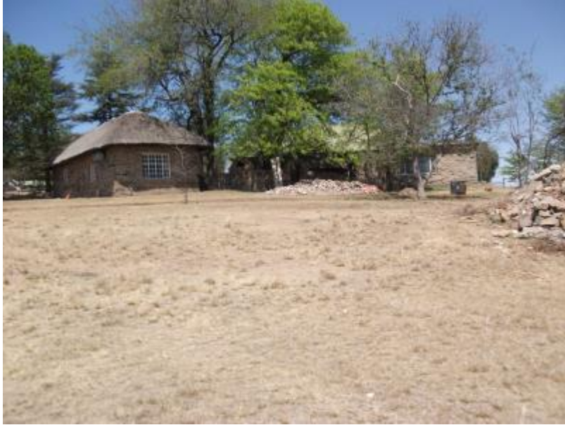
Figure 69: The main residence (FC02.1) (right) and an elongated outbuilding (FC02.1) which was constructed with the same material (left) (above). Note the dump with dresses and undressed dolerite stone suggesting that the complex of buildings was recently altered and upgraded (above).
