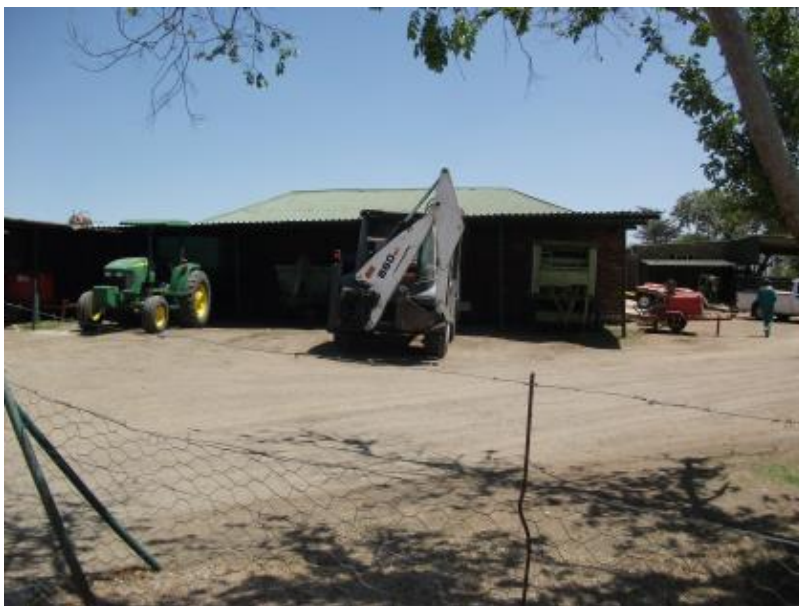
Figure 72: The shed complex (FC02.5) that is part of FC02 comprises several structures that were added to a main shed which was constructed with dolerite stone. The extended, plastered structures were constructed with clay bricks and perhaps with cement bricks as well. The fitted window and door frames were manufactured from steel (above).
