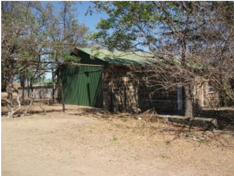
Figure 70: The second outbuildings in FC02 (FC02.1) has a near square ground plan and was constructed with dressed dolerite stone, fitted with steel window frames and steel door and is covered with a with pitched corrugated iron roof (above).
