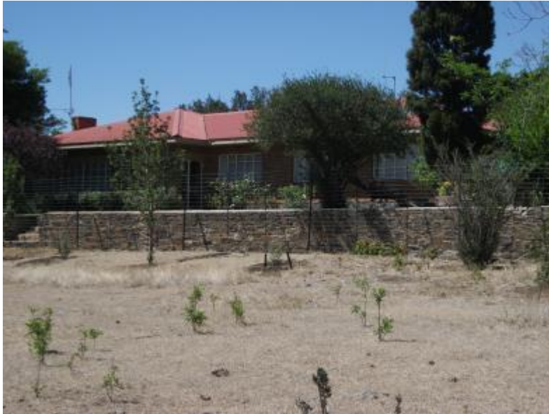
Figure 66: The main residence (FC01.1) in FCO1 comprises a multi-room dwelling which was built with clay bricks and fitted with a pitched corrugated iron roof and steel window frames (above).
