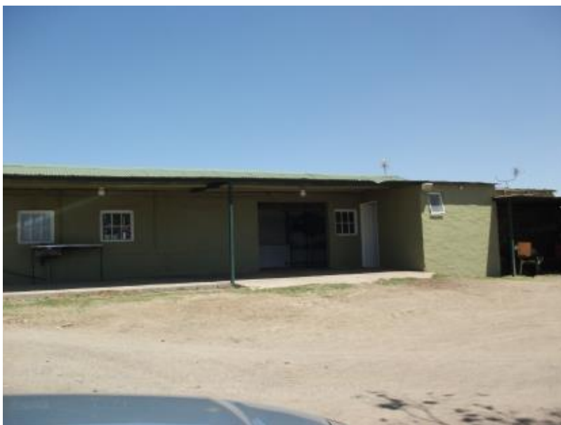
Figure 73: One of the extensions of FC02.5 was constructed with clay bricks and plastered with cement and is fitted with a low-pitched corrugated iron roof (above).
