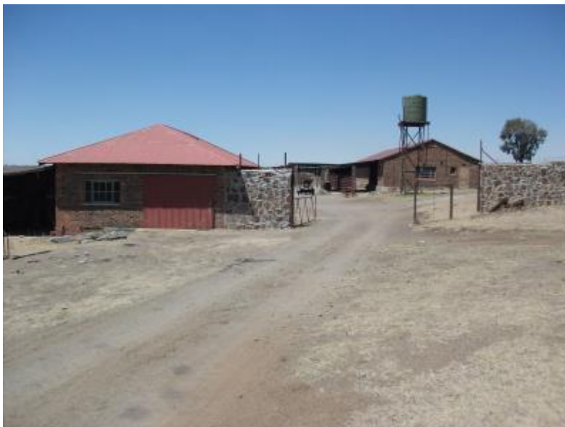
Figure 67: The two sheds (FC01.2, FC01.3) in FCO1 were both constructed with clay bricks and fitted with pitched corrugated iron roofs and steel window frames (above).
