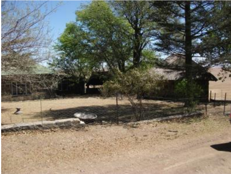
Figure 71: The rondavel (FC02.4) near the main residence. It was constructed with dolerite and fitted with a pitched grass roof (above).
