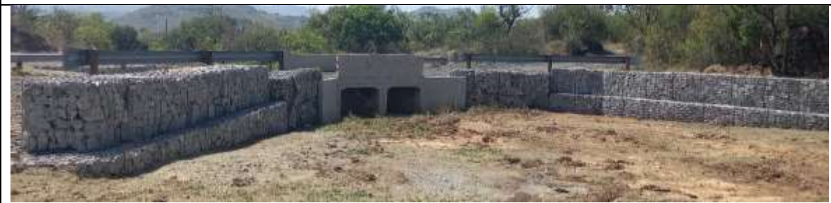
Plate 3.3: Culvert and gabion side walls of W1.1 road crossing
