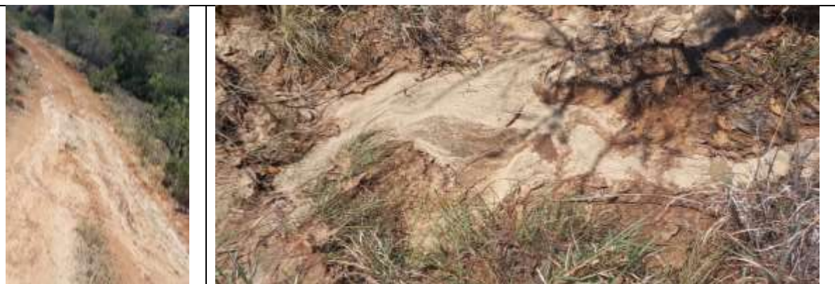
Plate 3.24: Access road crossing and downstream braided alluvial channel of W4.
