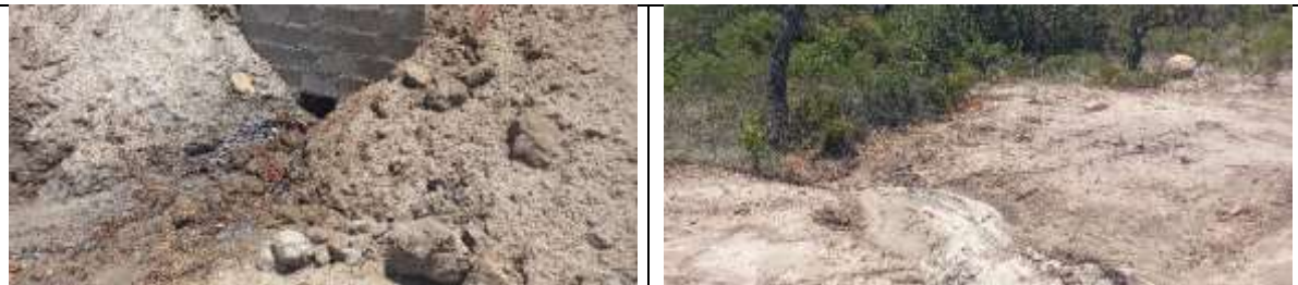
Plate 3.21: Small culvert, creating a knick point and downstream erosion and sedimentation.
