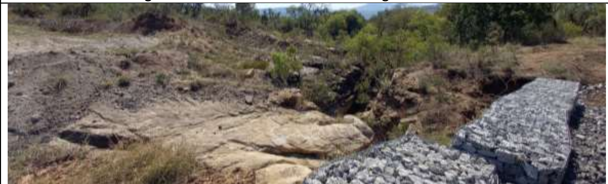
Plate 3.9: Downstream bedrock section of W1.1
