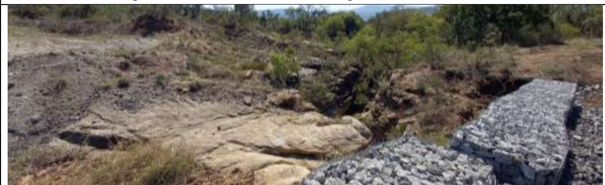
Plate 3.4: Downstream bedrock section of W1.1
