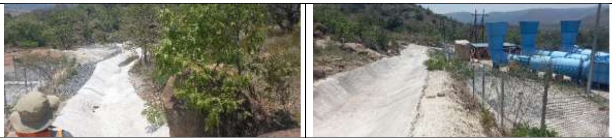
Plate 3.20: Concrete cut-off drain surrounding existing ventilation shaft and feeding into W1.11.
