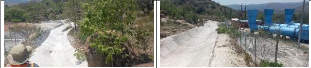
Plate 3.25: Concrete cut-off drain surrounding existing ventilation shaft and feeding into W1.11.
