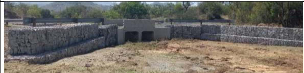
Plate 3.8: Culvert and gabion side walls of W1.1 road crossing
