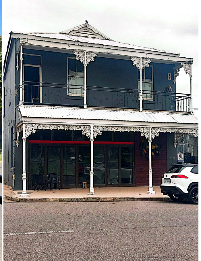
site photos of existing wrought iron balustrade 01/12/2022
