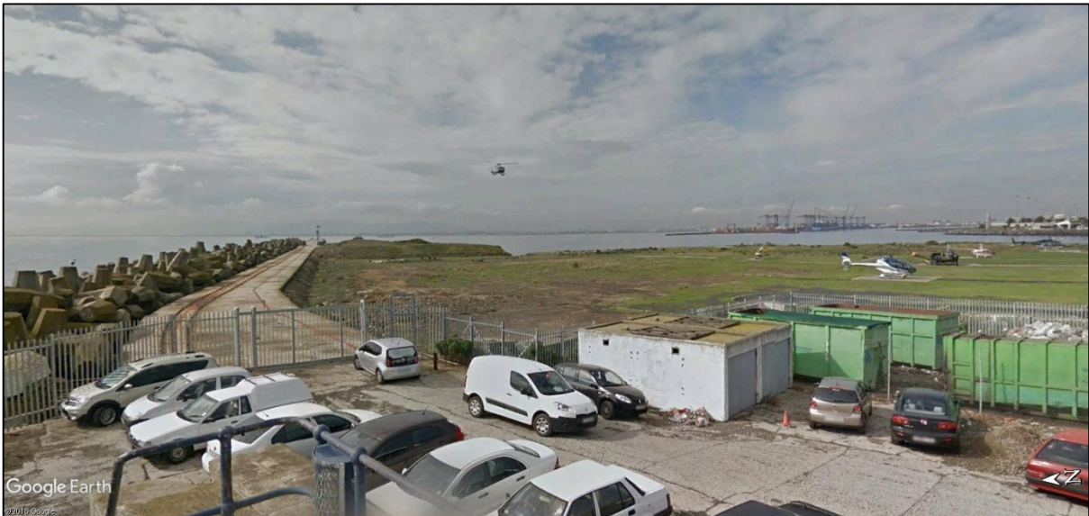
Photograph 4.11: Looking north-east from the terminus of the original seawall down the new portion of breakwater. The area located to the right of the breakwater was only reclaimed during the late 1990s. This area would accommodate the marine abstraction structure, pump house and portion of the raw water intake pipeline. The brine outfall would feed into the cap of the concrete portion of the breakwater structure, more or less at the bend in the structure (Source: Google Earth Street View, May 2015).
