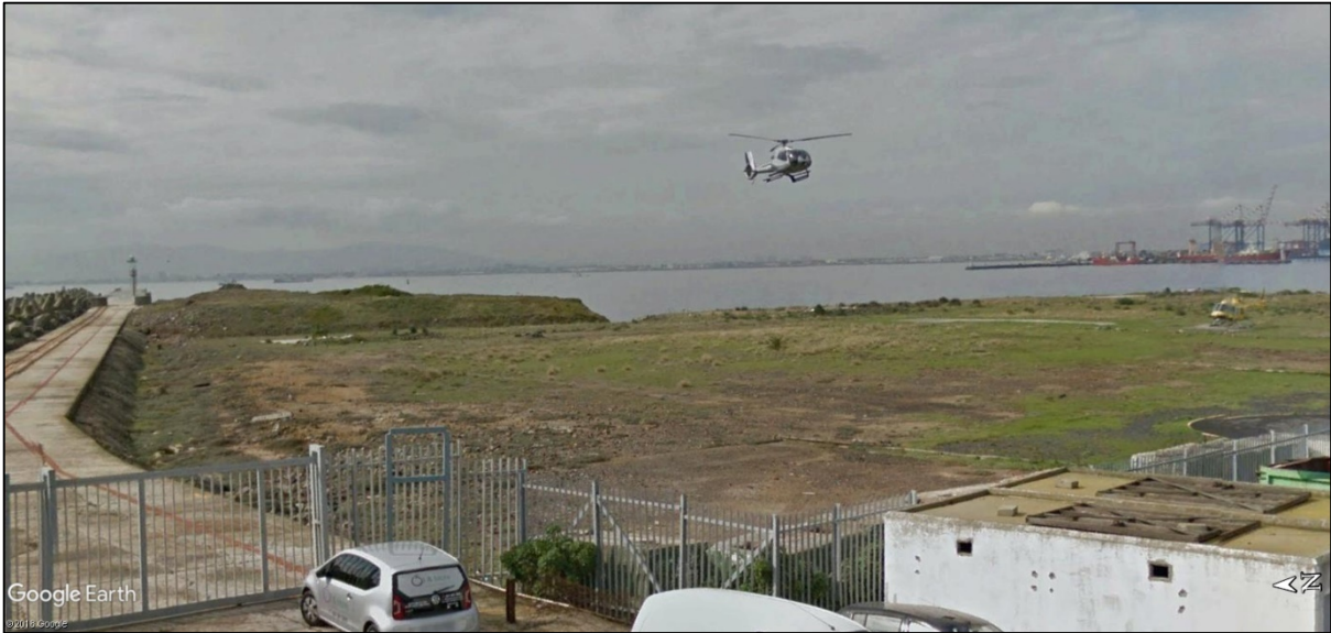
Photograph 4.12: Close-up of reclaimed area which would accommodate the marine abstraction structure, pump house and a portion of the raw water intake pipeline. The pumphouse would be located on the heli-pad on the right (white line in middle-distance) (Source: Google Earth Street View, May 2015).
