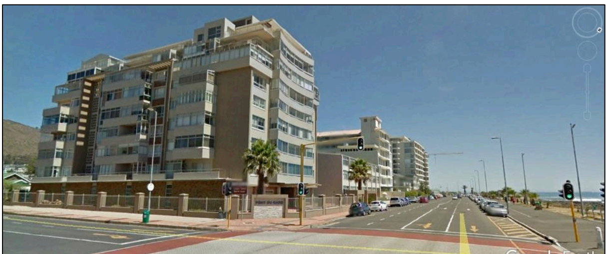
Photograph 14: Apartment blocks across Beach Rd from the western portion of the plant site, seen from the east of the intersection with Fritz Sonnenberg Rd. (Source: Google Earth Street View, March 2015).
