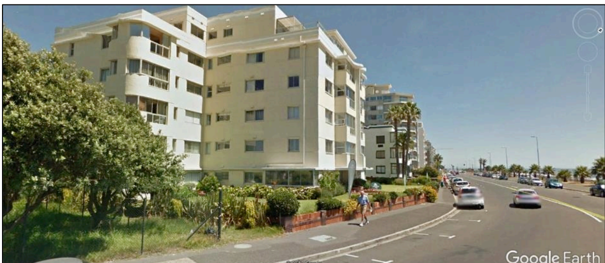
Photograph 23: Easternmost apartment block along Beach Rd, Mouille Point (opposite CPUT parking area), seen from the east. The raw water pipeline would be located on the pavement. (Source: Google Earth Street View, March 2015).
