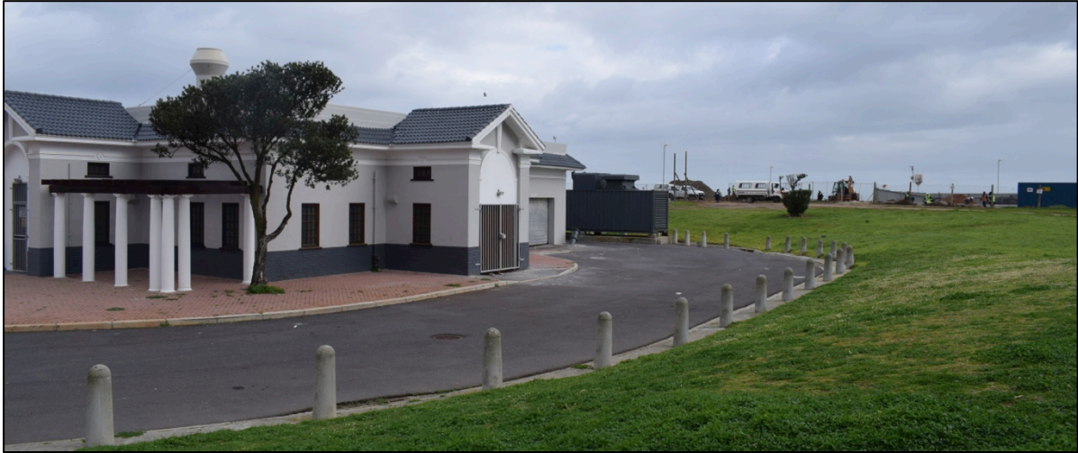
Photograph 3: Promenade Precinct 2 Pump station, 2017 The brine discharge pipeline would be connected to the station
