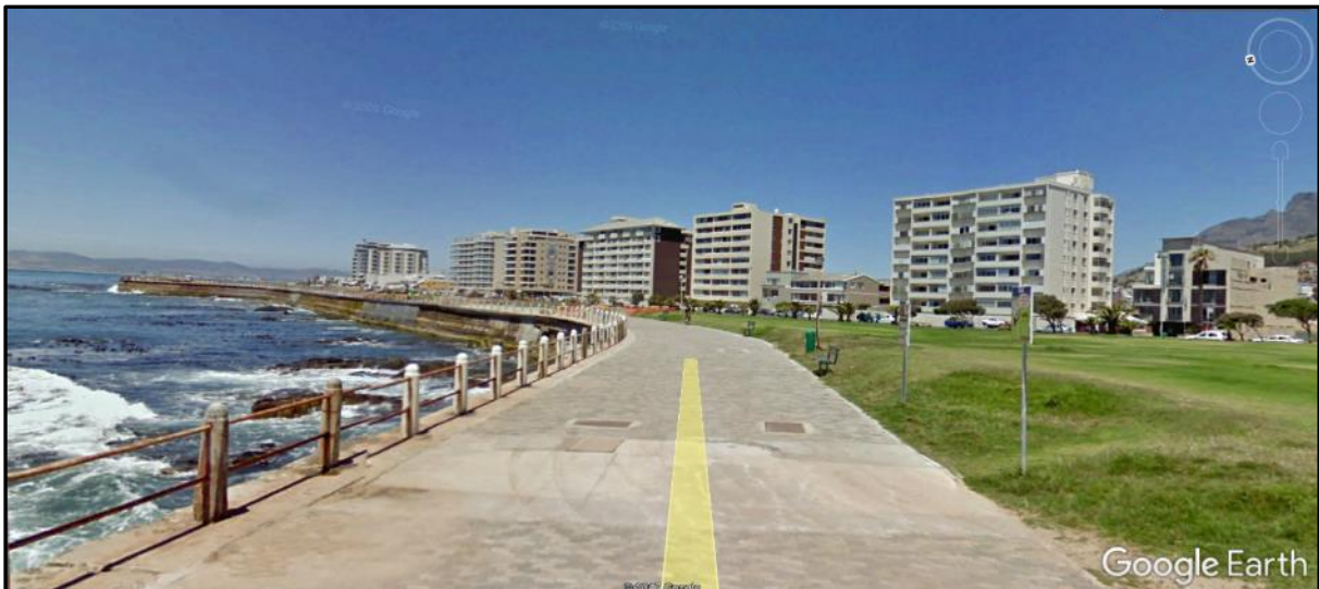
Photograph 4: Promenade and Sea wall east of the Green Point Lighthouse. The brine discharge pipeline is proposed to be aligned along the seawall. (Source: Google Earth Street View, March 2015).
