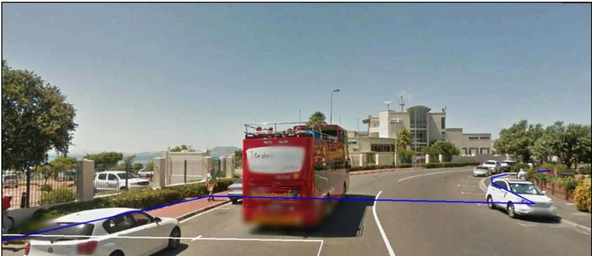
Photograph 22: Raw water intake pipeline (blue line) traversing Beach Road west of CPUT's Granger Bay Campus. (Source: Google Earth Street View, March 2015).
