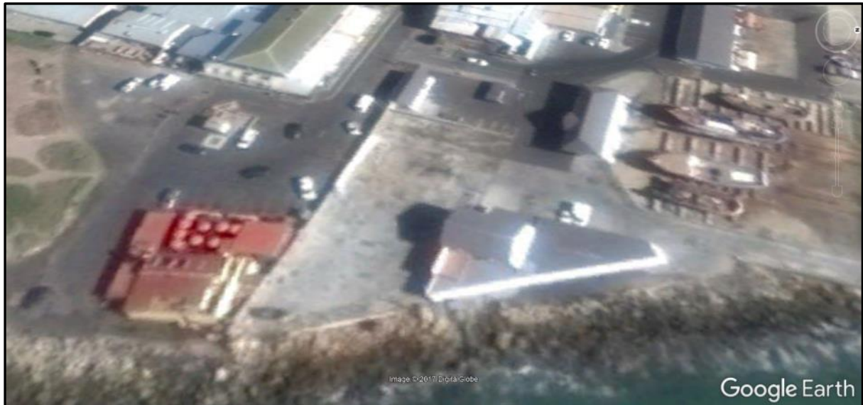
Photograph 11: Satellite image of raw water pump station site viewed from the east (Source: Google Earth 2017-07-27).
