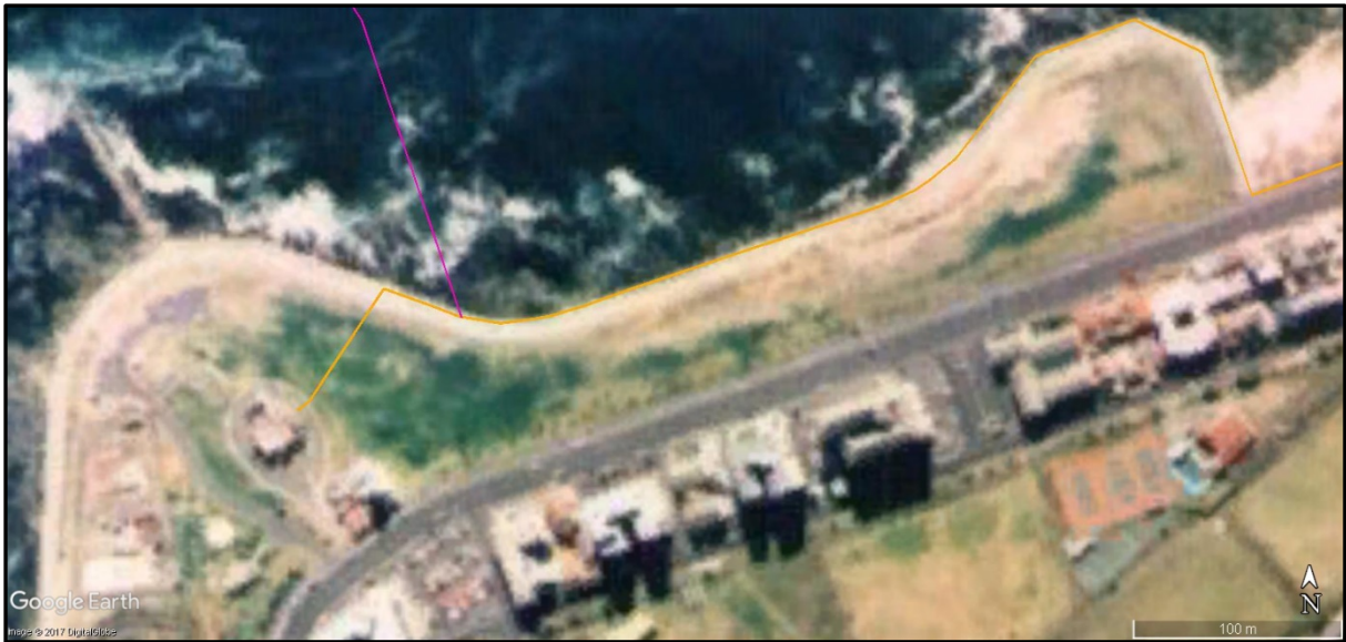
Figure 5.2.8: Terminal portion of brine discharge pipeline (orange line) and existing outfall (pink line) in local context.
