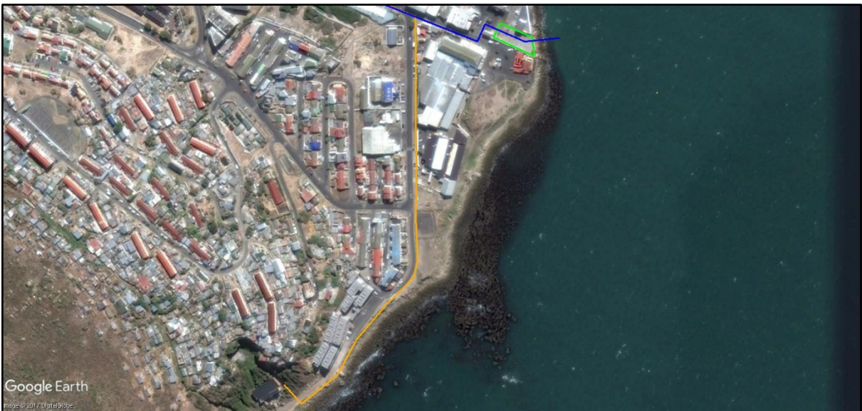
Figure 5.5.1: Raw water pump station site, raw water pipeline (including marine abstraction), and portion of brine discharge pipeline in local context 2017. (Source: Google Earth, 2017-05-12).
