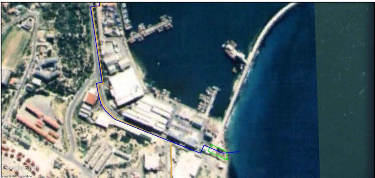
Figure 5.3.5: Raw water pipeline (including marine abstraction), raw water pump station site, and portion of brine discharge pipeline in local context 1996. (Source: Chief Directorate National Geo-spatial Information. 994/96_01N_00001).
