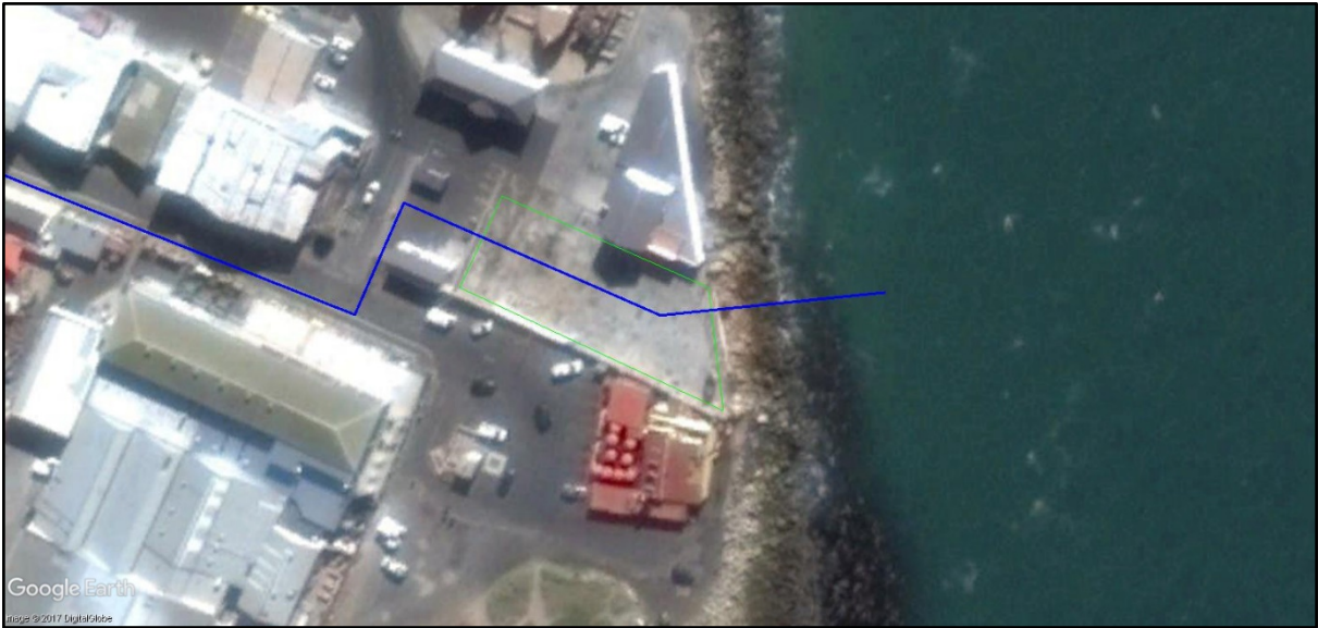
Figure 5.4.8: Raw water pump station site and raw water pipeline (including marine abstraction) pipeline in local context 2017. (Source: Google Earth, 2017-05-12).
