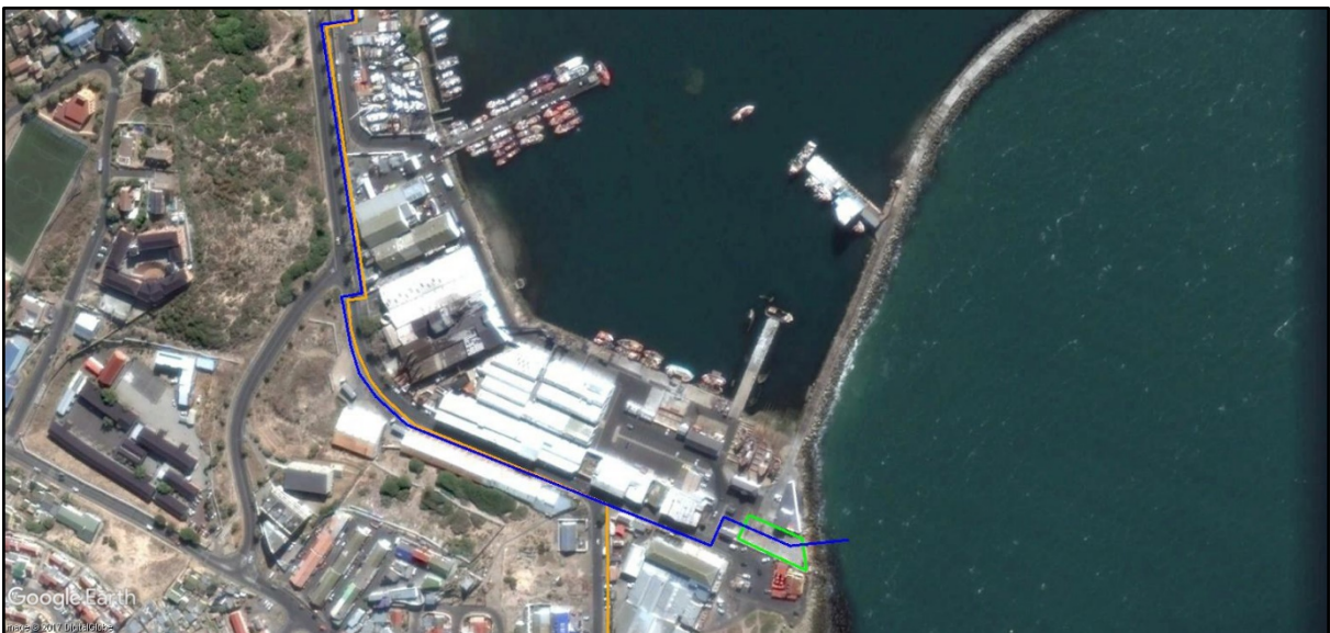
Figure 5.3.1: Raw water pipeline (including marine abstraction), raw water pump station site, and portion of brine discharge pipeline in local context 2017. (Source: Google Earth, 2017-05-12).
