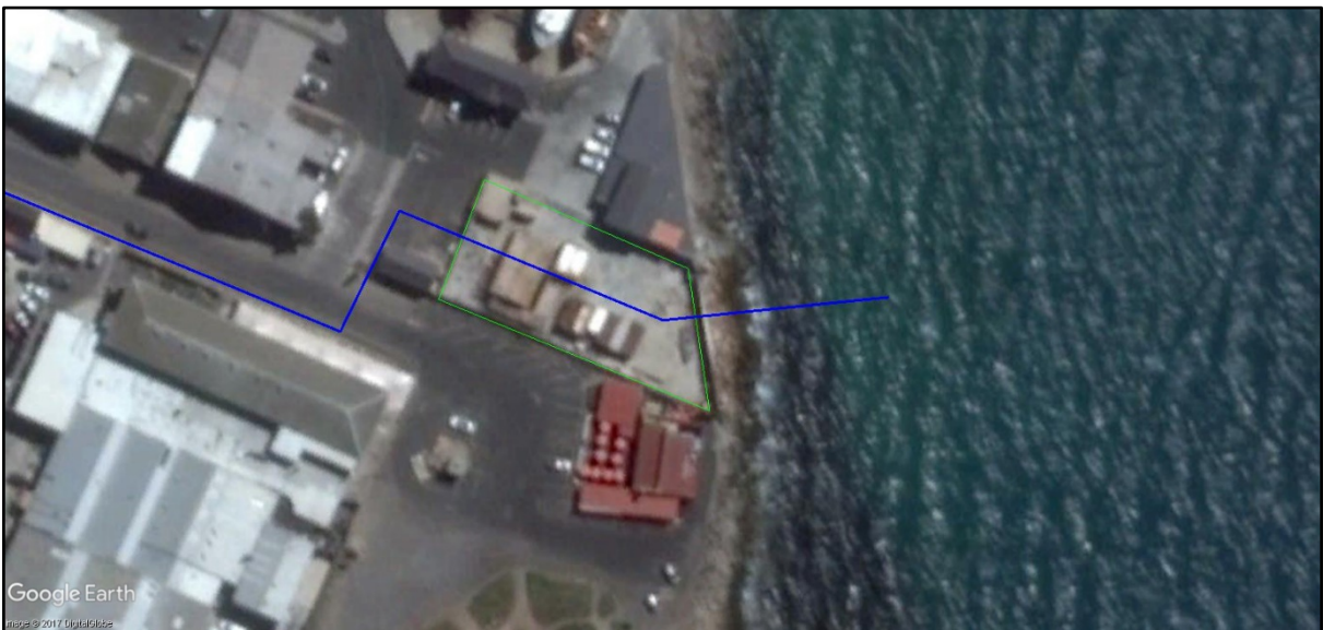
Figure 5.4.8: Raw water pump station site and raw water pipeline (including marine abstraction) pipeline in local context 2014. (Source: Google Earth, 2014-02-25).
