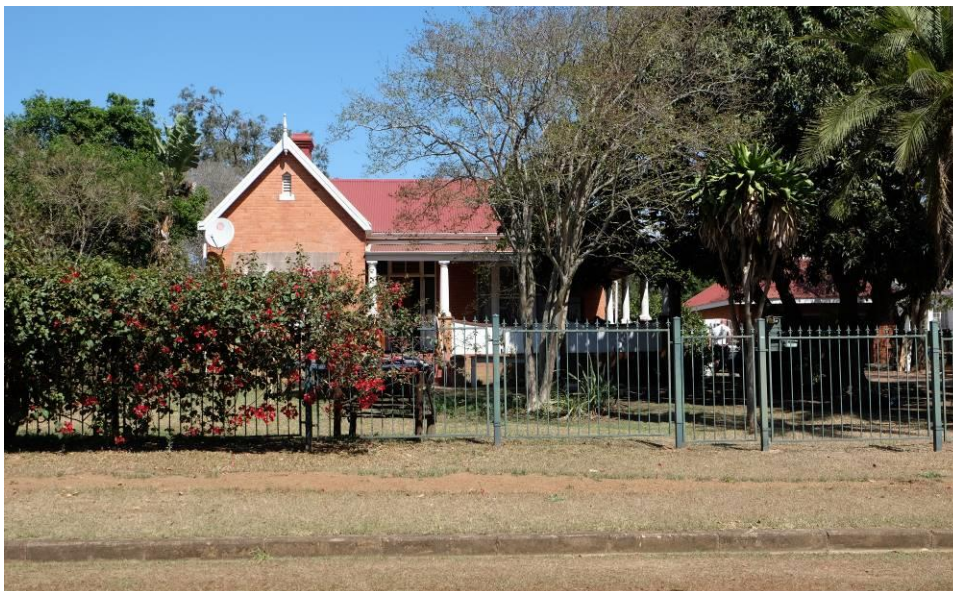
Fig. 7_Street elevation with main entrance to Roseveare Road, single storey red brick and corrugated roof residence with triangular gable and corner verandah supported by columns (Source: tsica heritage consultants, 22.09.2020)
