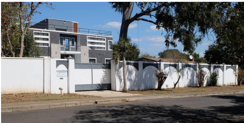
Fig. 60_View along Carbis Road in western direction with newly built double storey residence (Source: tsica heritage consultants, 22.09.2020)
