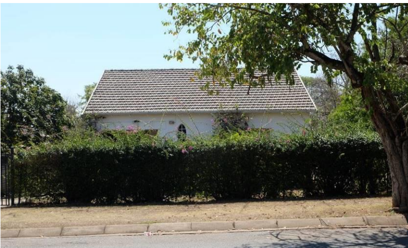
Fig. 66_ Single storey tiled roof residence from around 1930s along Carbis Road (Source: tsica heritage consultants, 22.09.2020)
