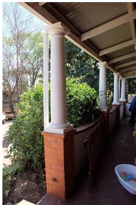
Fig. 16 & 17_Verandah wrapped around the corner (left); Verandah roof is supported by a row of columns (right) (Source: tsica heritage consultants, 22.09.2020)
