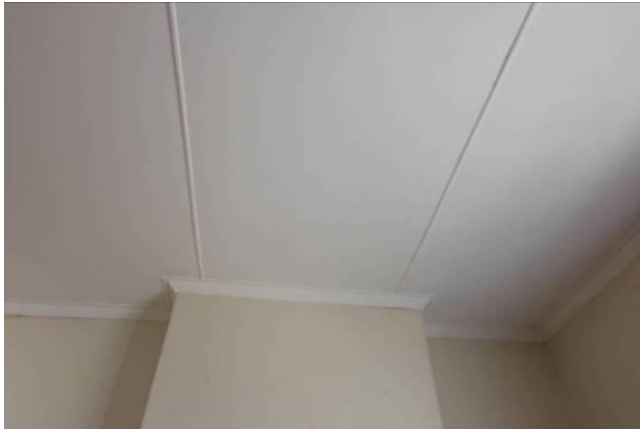
Fig. 38_Original ceiling boards in lounge area (Source: tsica heritage consultants, 22.09.2020)
