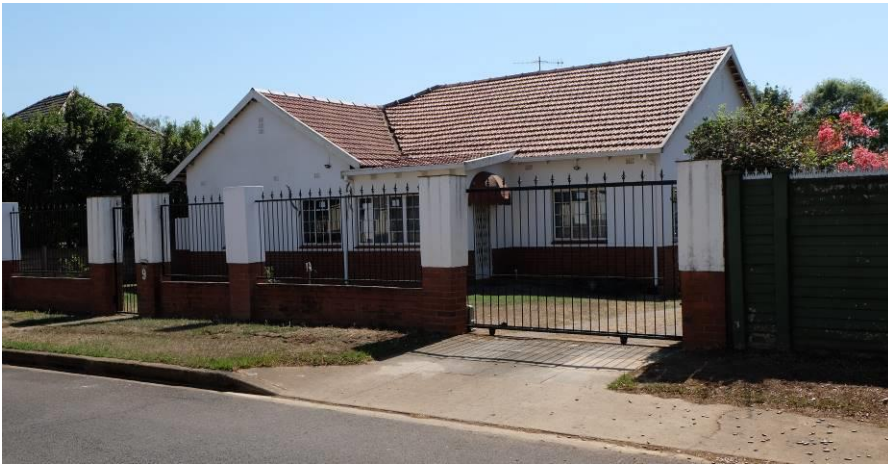
Fig. 64_ Typical single storey tiled roof residence from around 1950s along Roseveare Road (Source: tsica heritage consultants, 22.09.2020)
