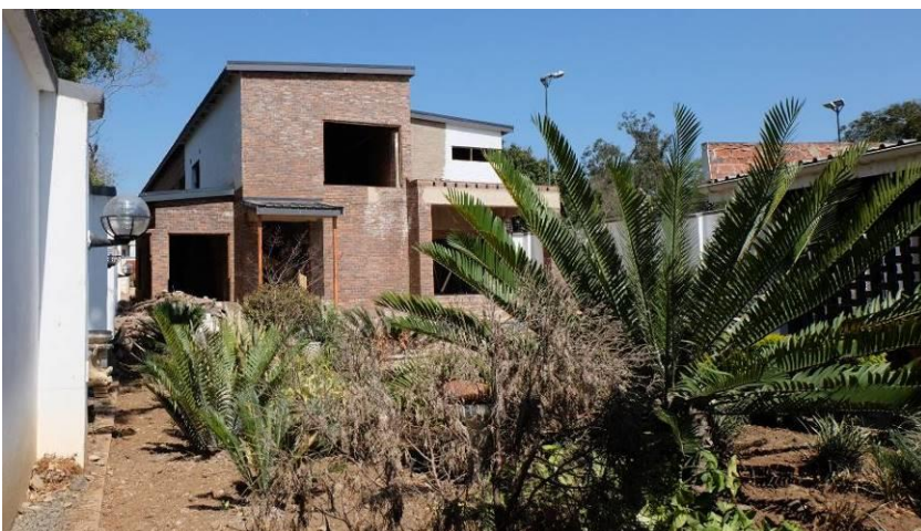
Fig. 63_New double storey development along Carbis Road (Source: tsica heritage consultants, 22.09.2020)
