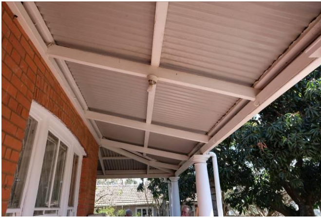
Fig. 19_ Verandah roofing with wooden trusses (Source: tsica heritage consultants, 22.09.2020)
