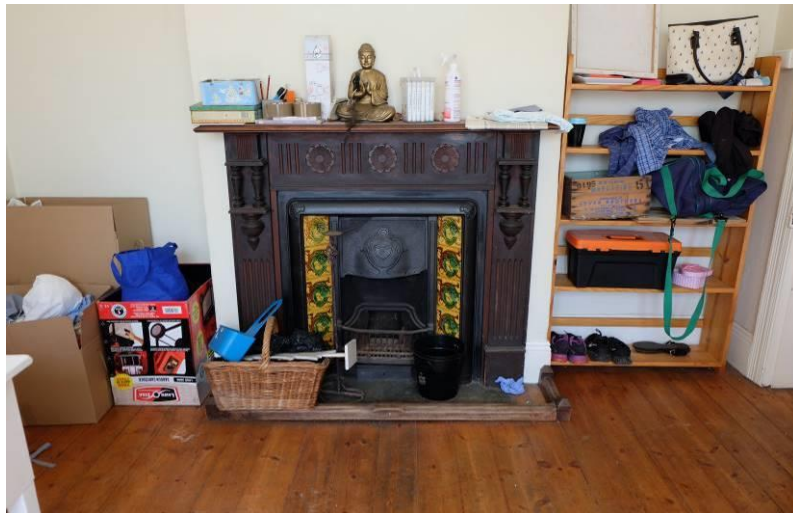
Fig. 35_Original fireplace and wooden floor boards in bedroom (Source: tsica heritage consultants, 22.09.2020)
