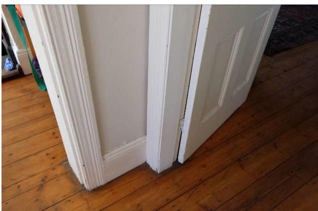
Fig. 41_Original wooden skirtings and door frames in most of the rooms still in good condition (Source: tsica heritage consultants, 22.09.2020)
