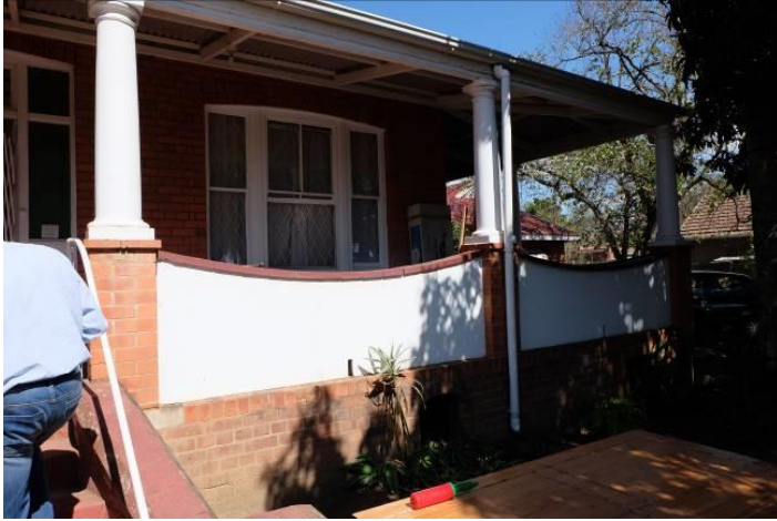
Fig. 15_Verandah roof supported by columns (Source: tsica heritage consultants, 22.09.2020)
