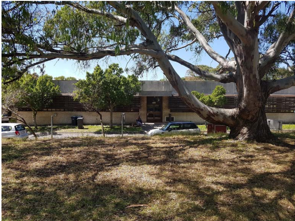
Photo 8: Technical Building (west facing elevation)
