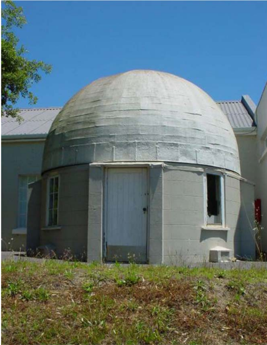
Photo 9: Heliograph (east facing elevation)
