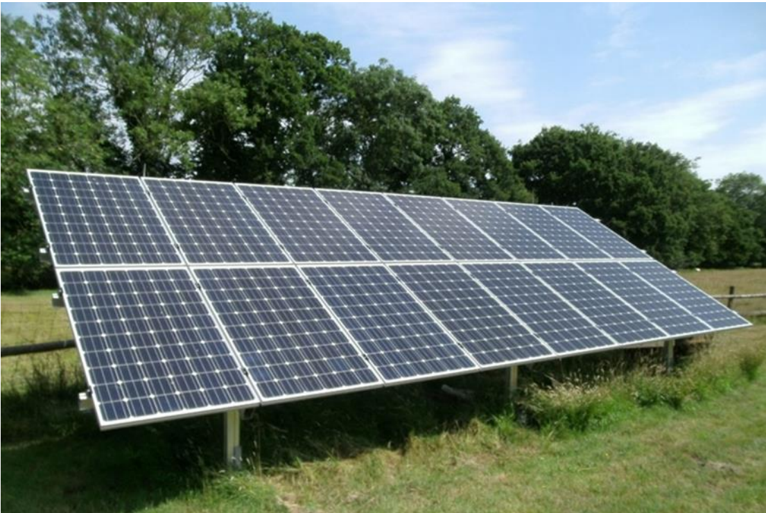
Figure 1.3: Stationary solar PV panels.
