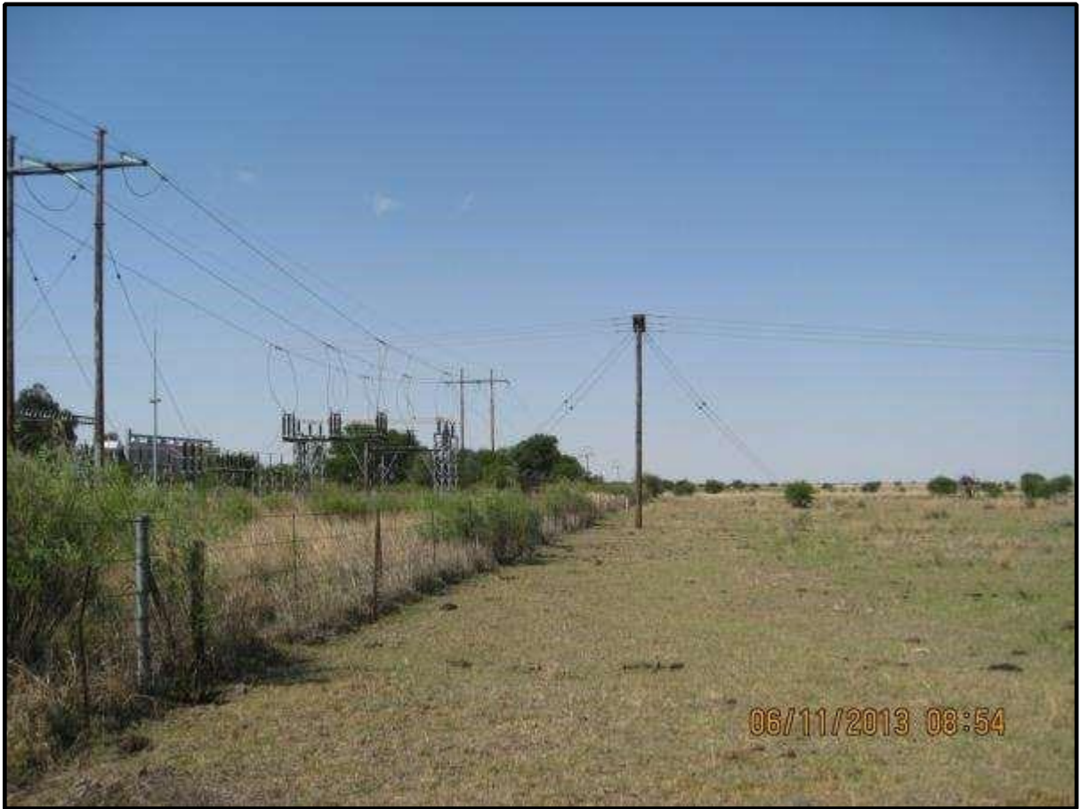
Photograph 1.4: View across PV site from the north with Heuningspruit substation on the left
