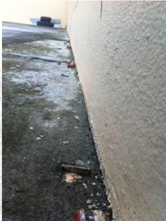
Signs of piping that ran along the wall
