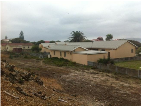
View from the South
