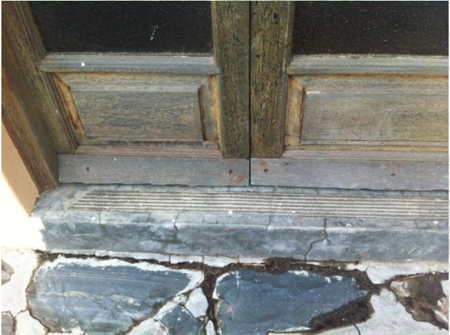
Details of cracked cement and rusting door handles
