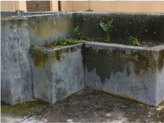
Wall running around the house and car entrance/driveway
