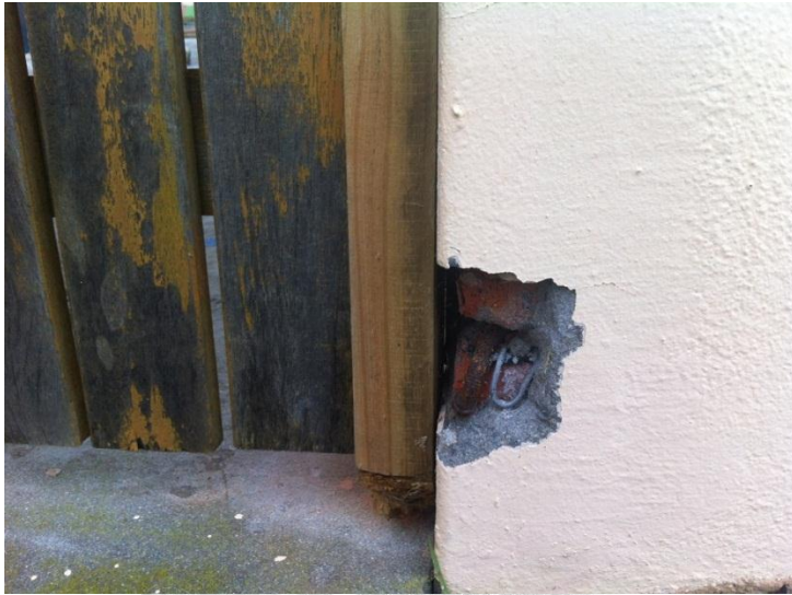
Cracking plaster
