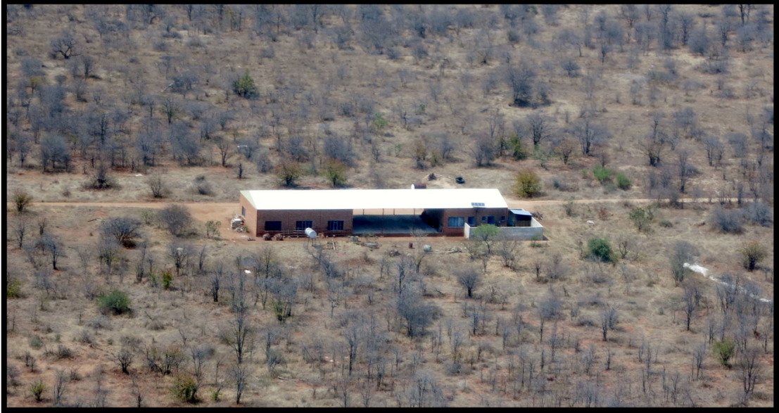
Photo 1: Typical site infrastructure – existing sheds and stores
