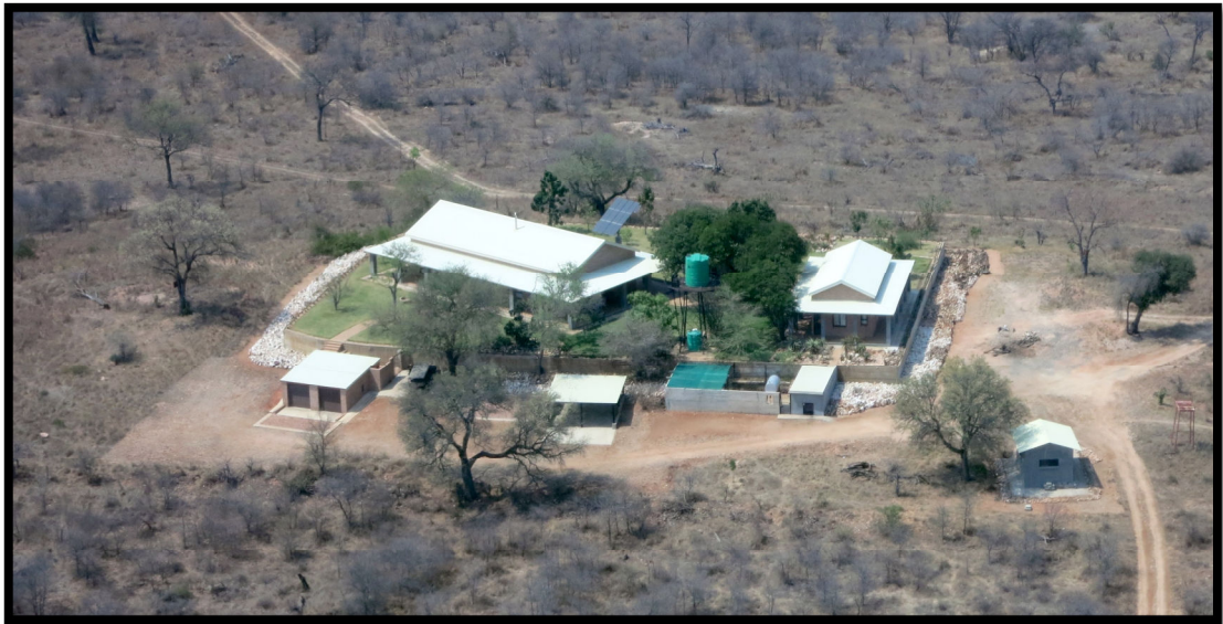
Photo 2: Typical site infrastructure – existing Rietvley farmhouse
