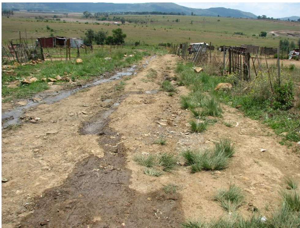
Figure 24: Typical sewage leak and dirt road observed within study area during the November 2017 assessment
