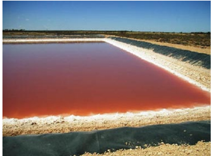
Figure 3: Example of wastewater evaporation pond
