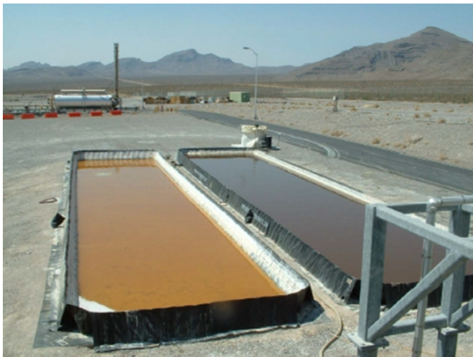
Figure 2: Example of wastewater evaporation pond
