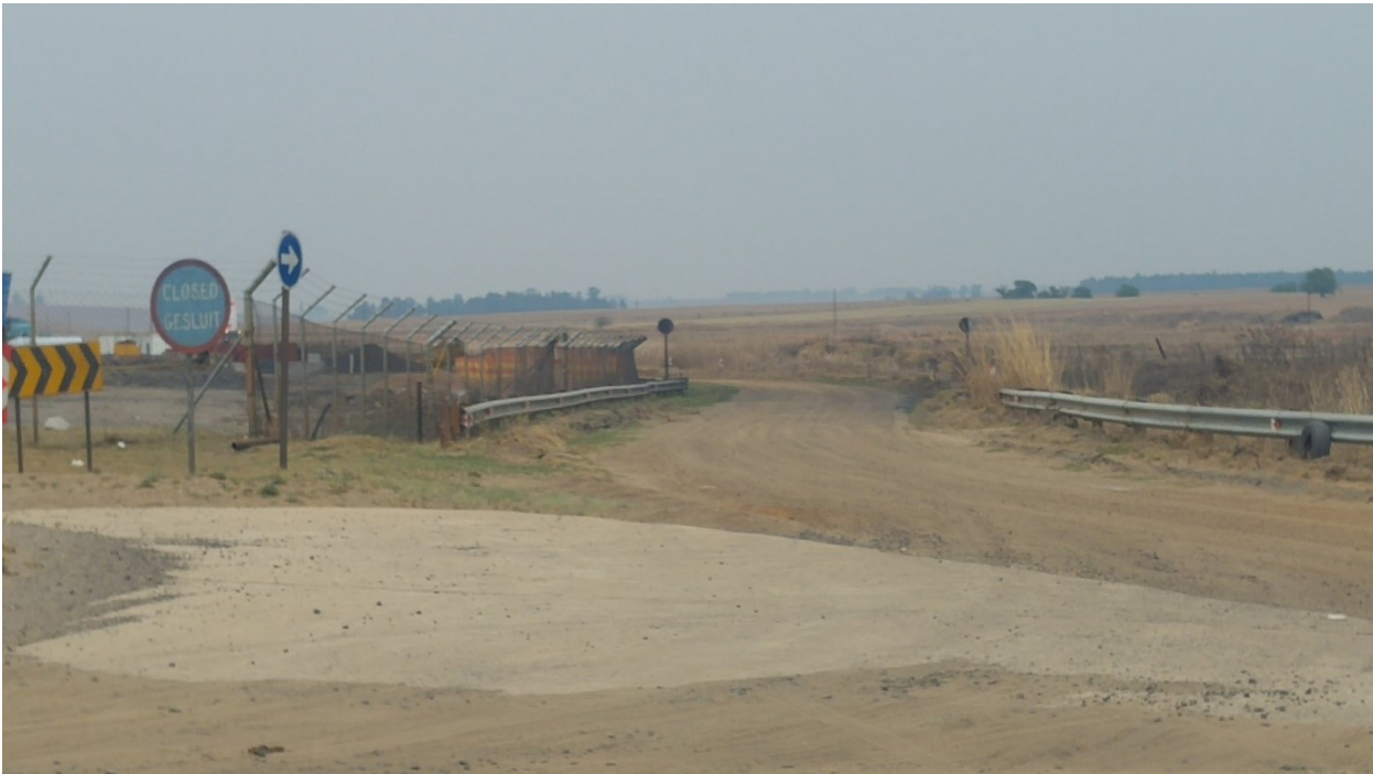
Photo 2: Realignment of and incorrect signage on public road D638
