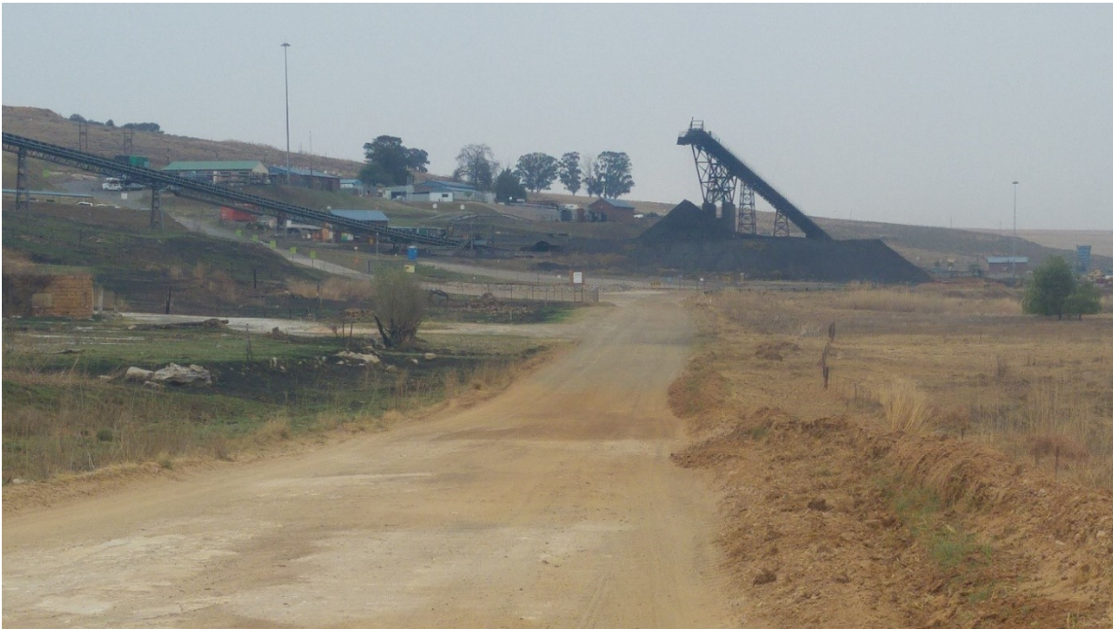
Photo 3: Main Access Road D638 at mine entrance
