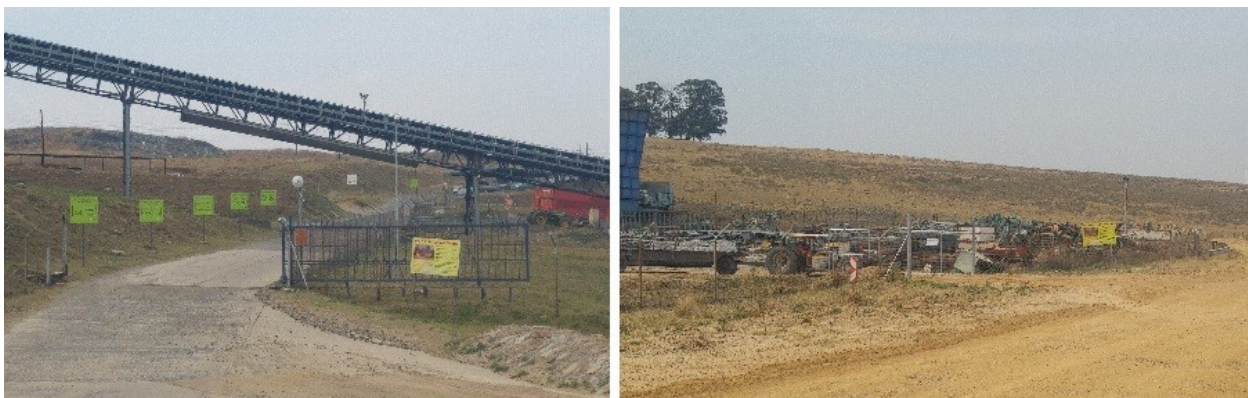
Photo 1: Main Access Gate (Left) and Maintenance Gate (Right)
