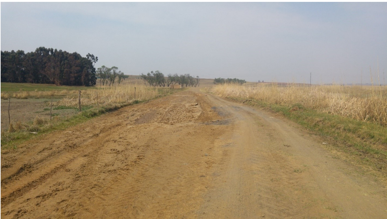
Photo 6: Secondary Access Road D638 south of the mine complex
