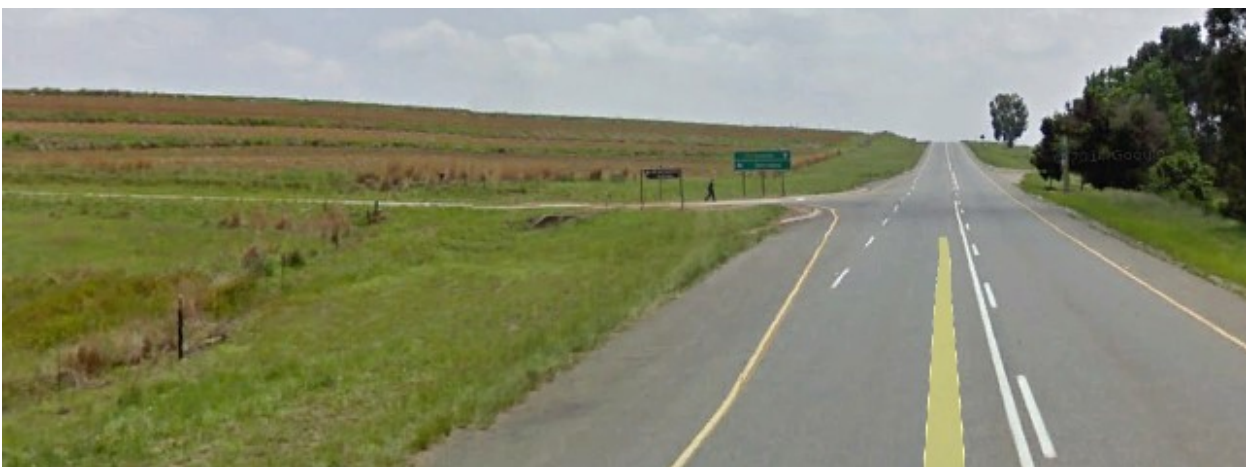
Photo 8: T-junction of secondary dirt access road D638 with R38
