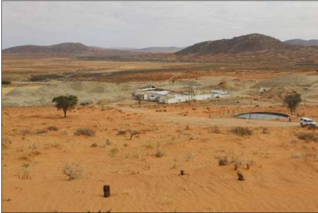
Figure 12. A broken building complex where the mine administration was based
