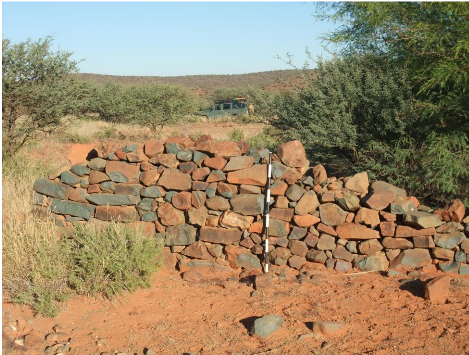
FIGURE 20: STONE WALLING IN DRY RIVER BED.
