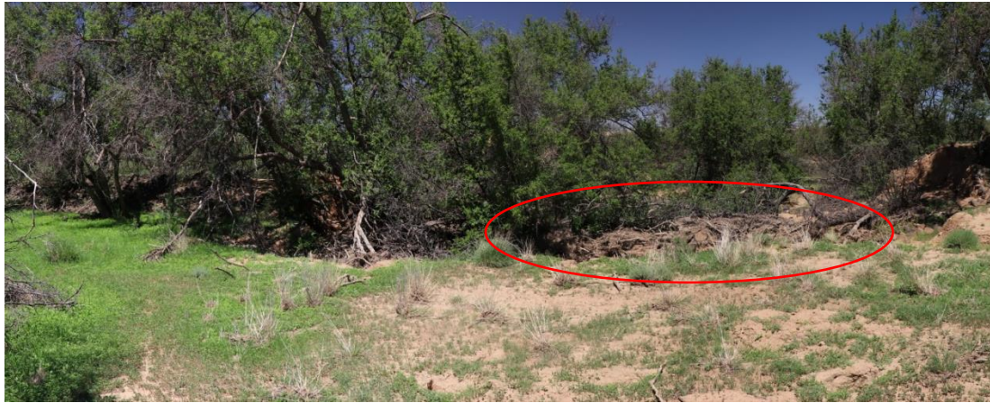
Figure 36: View of one of the small impoundments in the upper reach of the stream. The damwall has been breached and it is no longer functional. Note the large amount of flood debris (red) which should indicate that large water volumes are discharged during flash flooding.
