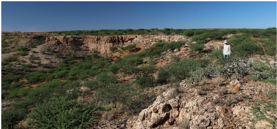
Figure 20: View of the calcrete cliff. Note the cliff height varies considerably.
