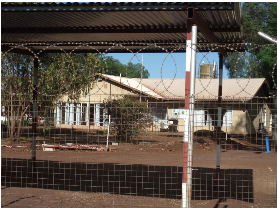
FIGURE 9: THE OFFICE COMPLEX. THIS IS AN OLD ASBESTOS FARM BUILDING. IT MAY BE OLDER THAN 60 YEARS BUT HAS NO INTRINSIC CULTURAL SIGNIFICANCE.
