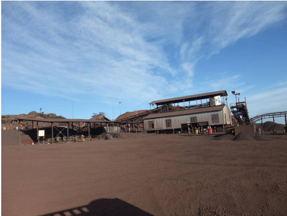
FIGURE 8: THE PLANT AREA.
