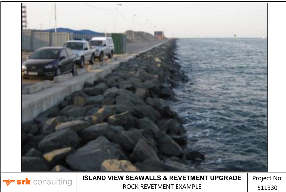
Figure 4-1: Example of a rock revetment
