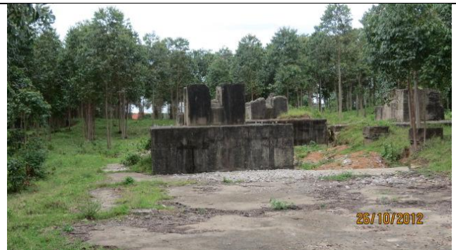
Relic foundations of the sawmill located within the eucalypt plantation.
