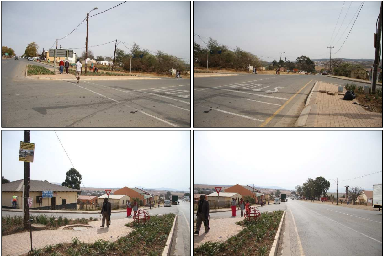
Plate 1: Intersection between the N2 Freeway and the R405 (towards Matatiele), within the town of Mount Frere. Also, the start of the road section under investigation.
