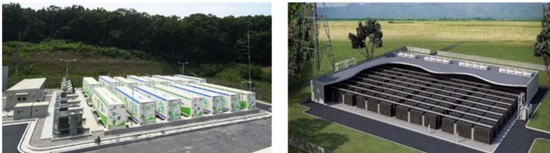
Figure 3: typical configuration of BESS installed inside containers and buildings
