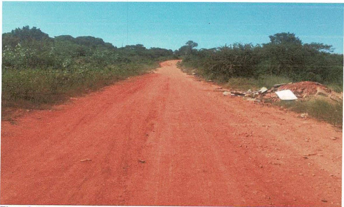
Figure 2: View of the southern section of the proposed area for construction.
