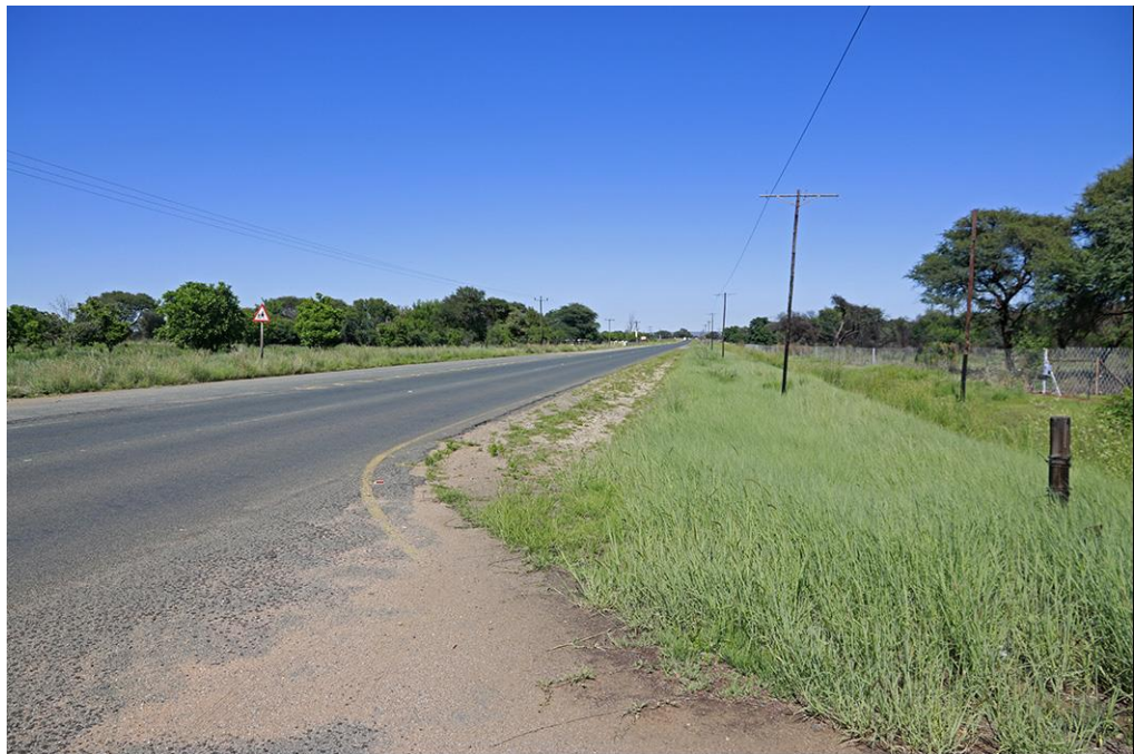
Photo 4: Sight distance to the west
