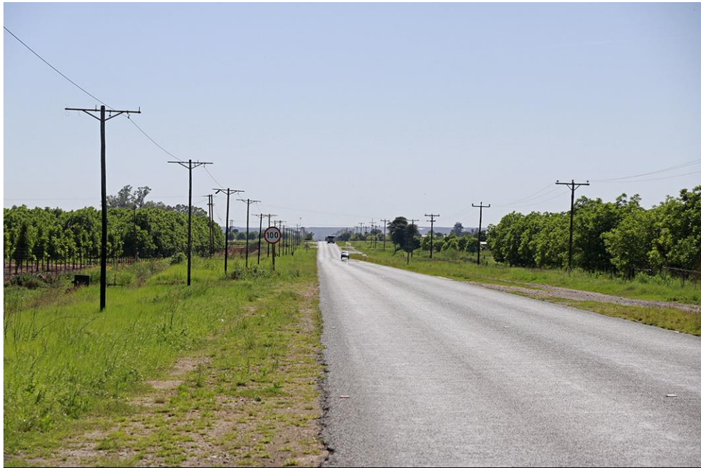
Photo 1: Road as seen towards Hartswater
