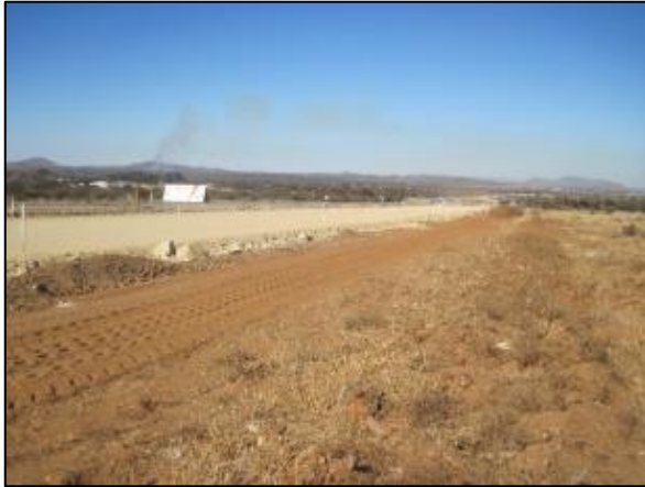
Figure 3: View of the N1 eastern bypass under construction.
