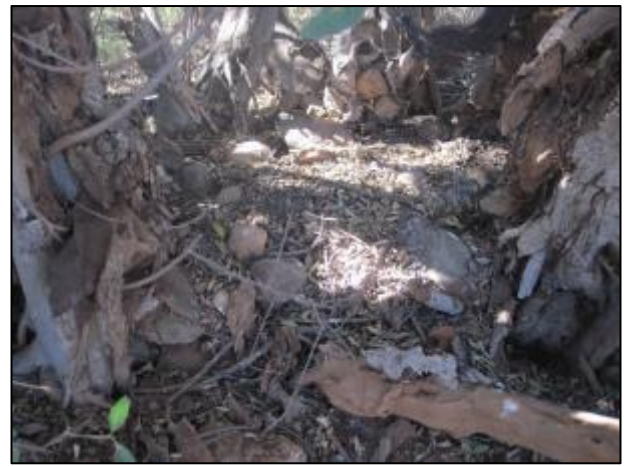
Figure 14: Close up view of the packed stone wall at site LIM 003.
