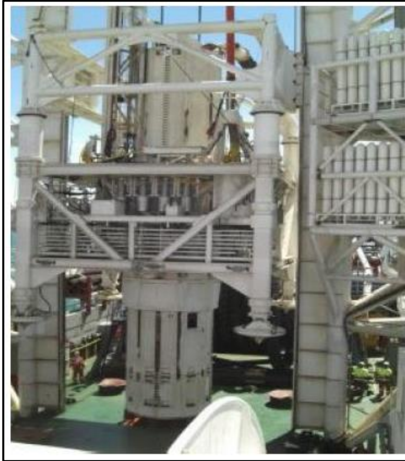
Figure 6: Example of the 2.5 m diameter drill bit within the drill frame structure
