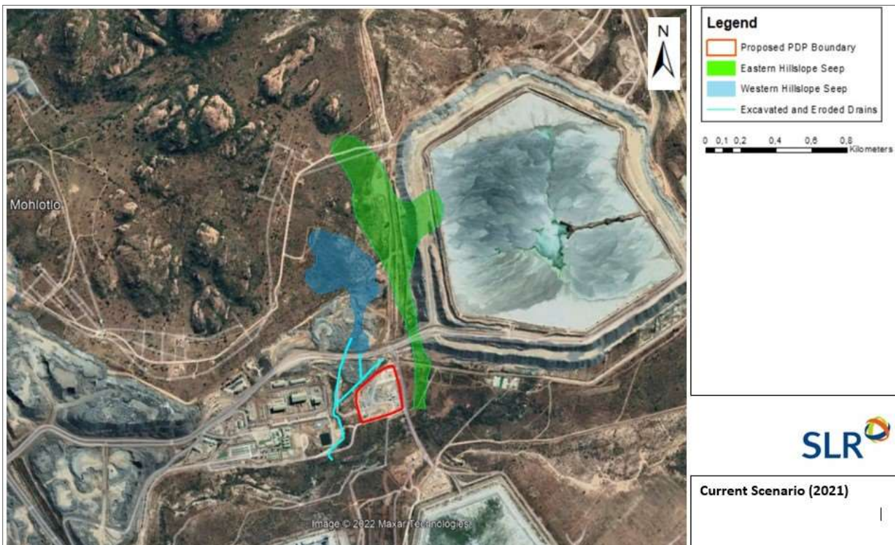
Figure 5.4: Extent of mining development surrounding the development site. The hillslope seeps are historic, the image illustrates the extent to which the mining operational area has encroached into them.
