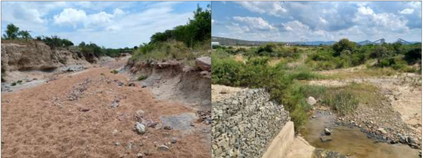
Figure 6.1: Channel incision, lateral scouring and sediment deposition in the Mohlosane River upstream of the study site (left); and lateral erosion and sediment deposition further downstream adjacent to the study site (right) (Photos- D. McCulloch).
