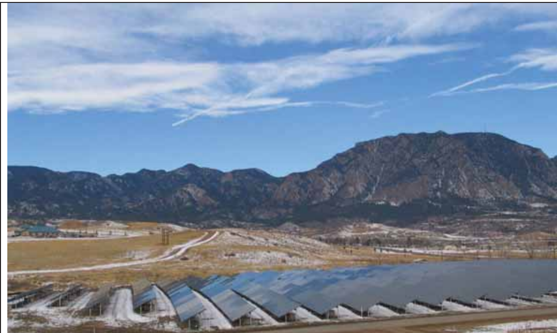
A 2-megawatt, ground mounted PV array occupies the site of a former landfill at Ft. Carson, Colorado, USA (Source: www.wapa.gov )
