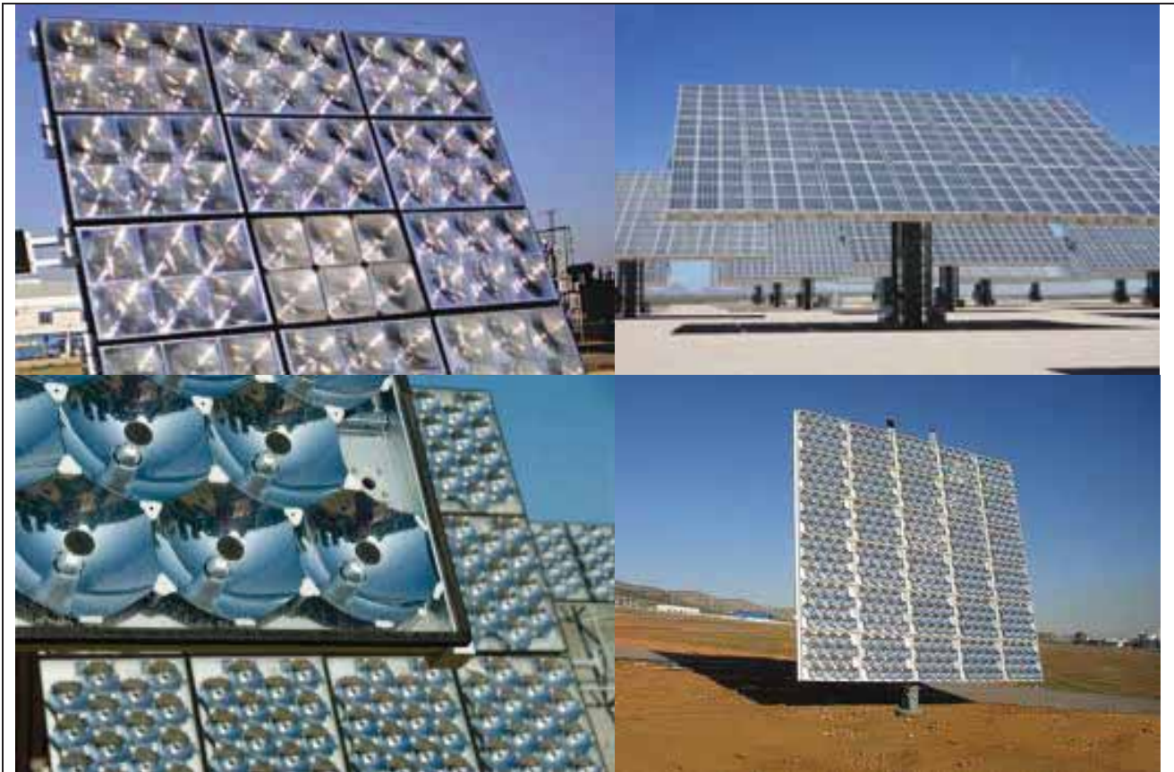
Figure 3-3: Example of Concentrated Photo-voltaic technologies (Bullis, 2011).
