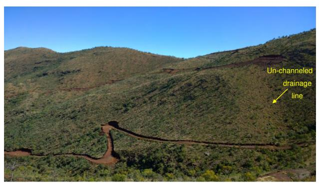
Figure 55: Prospecting road crossing an un-channeled drainage line.
