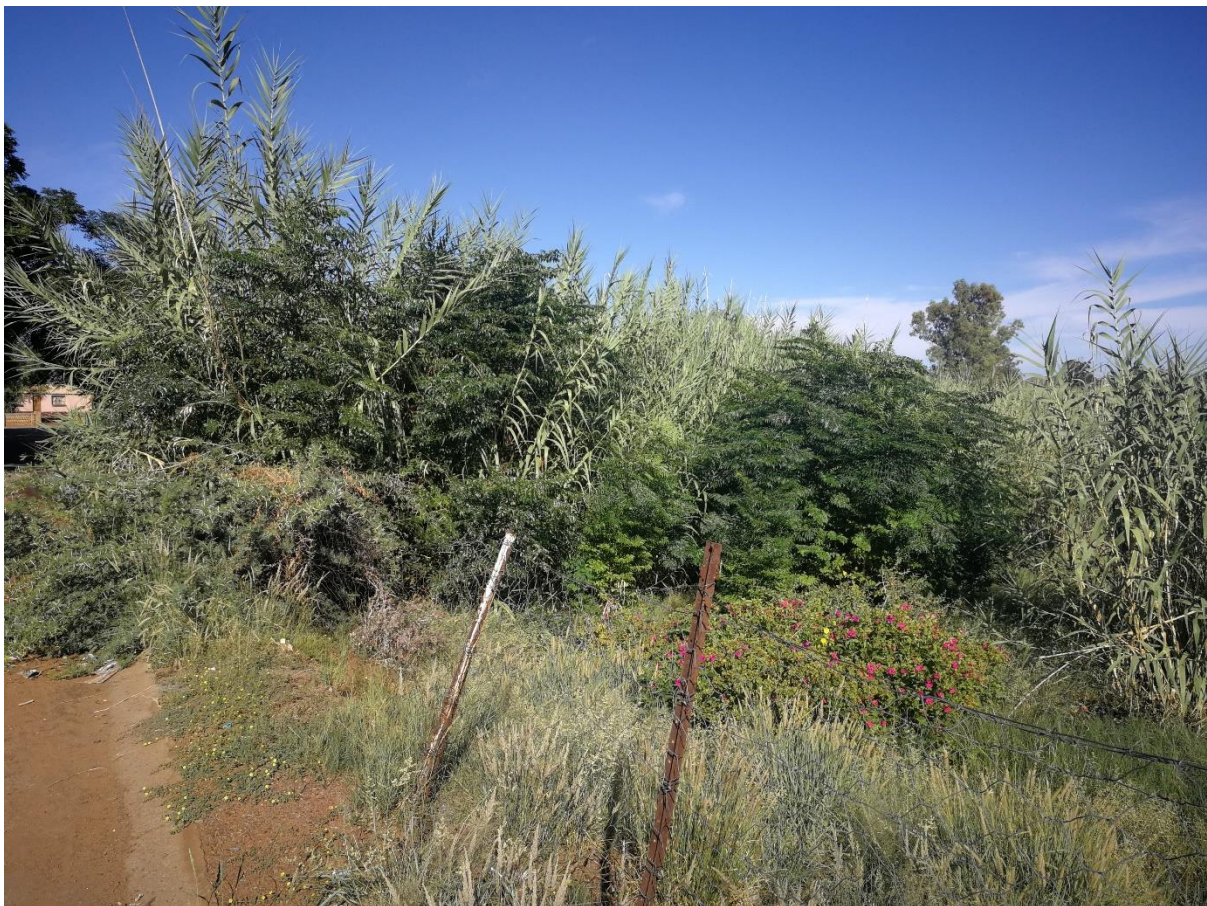
Photo 49: D41L-02299 flowing underneath Mossie Street in Wrenchville. Severely overgrown and disturbed. Direction: South-West
