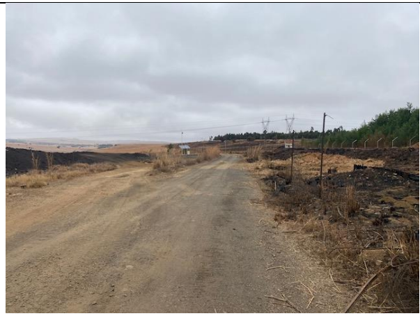
Access road to the Plan, with the Manganese Slag Stockpile on the left and the plant area on the right.
