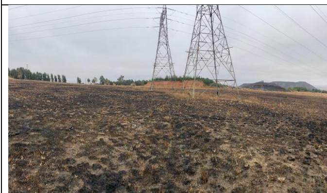
The proposed Plant is planned in the area of the topsoil stockpile.
