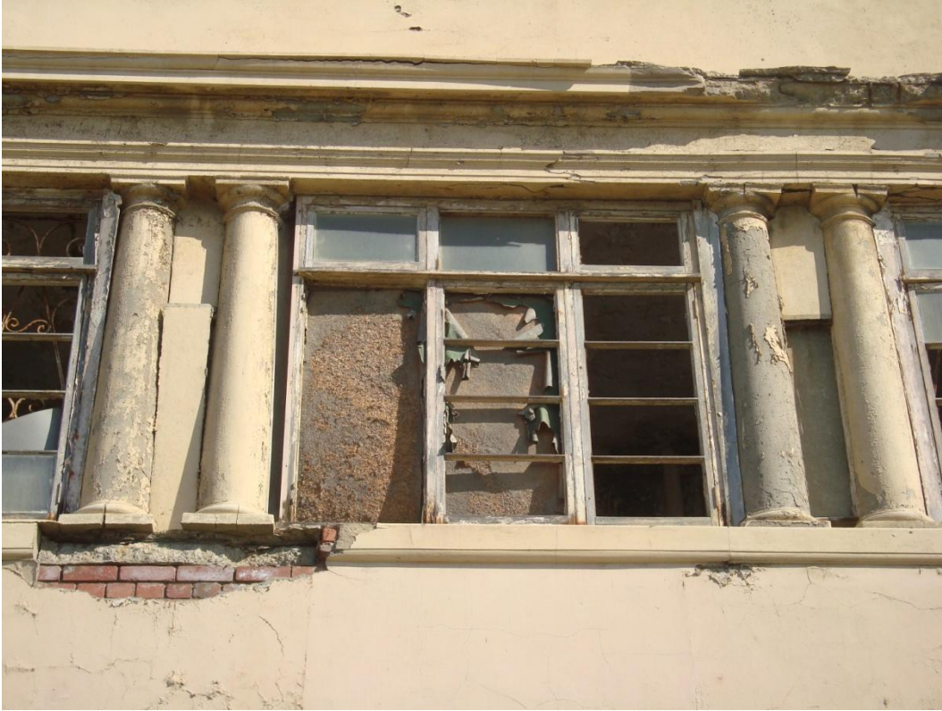
Figure 2 Window frame over East facade
