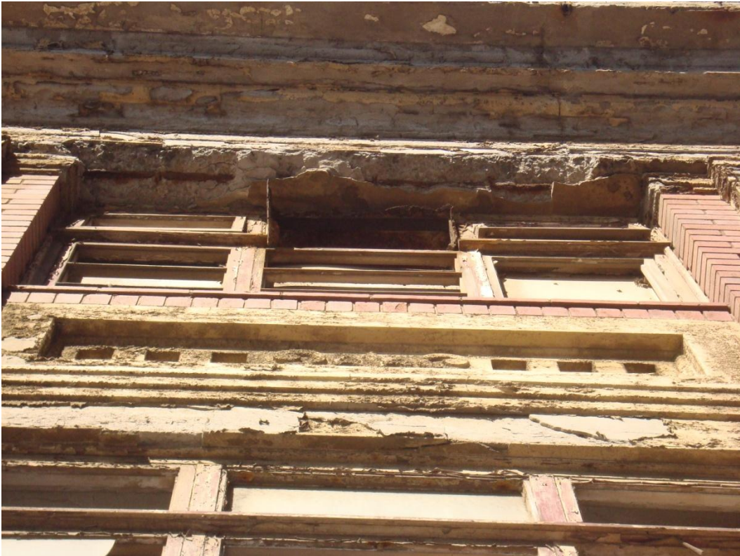
Figure 3 Roof ring beam on North facade
