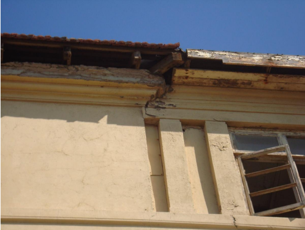
Figure 4 Roof ring beam on East facade
