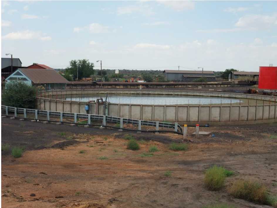
Figure 4: General view of the impacted area.
