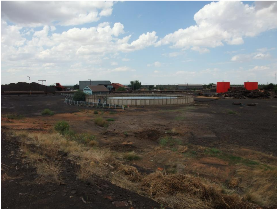
Figure 5: View indicating the disturbance.
