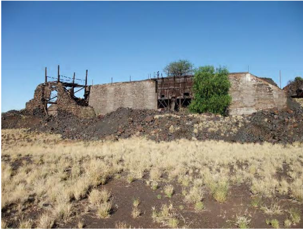
Figure 22: Old shoot used for ore transfer from coco pans to trucks or wagons.
