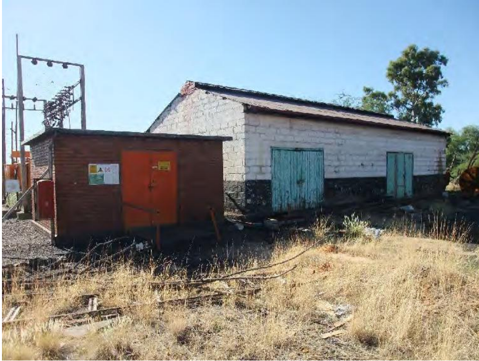
Figure 21: Old power station.
