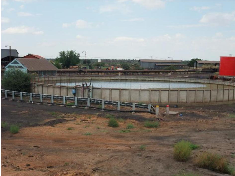
Figure 4: General view of the impacted area.
