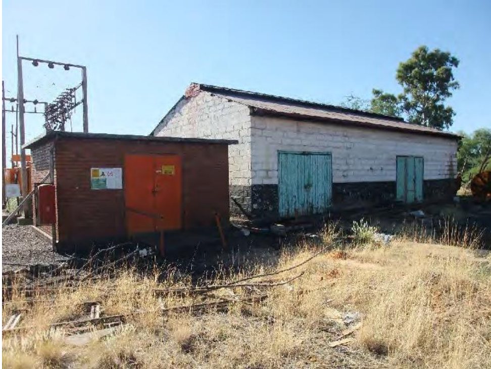
Figure 21: Old power station.
