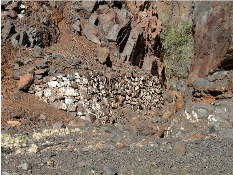
Figure 10: Stone wall with white wash used as stabilization.
