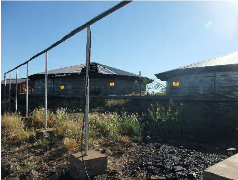
Figure 19: Water reservoirs on Black Rock koppie.
