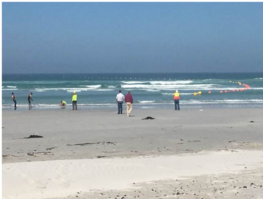
Figure 7 Cable being guided to shore by divers and small boats
