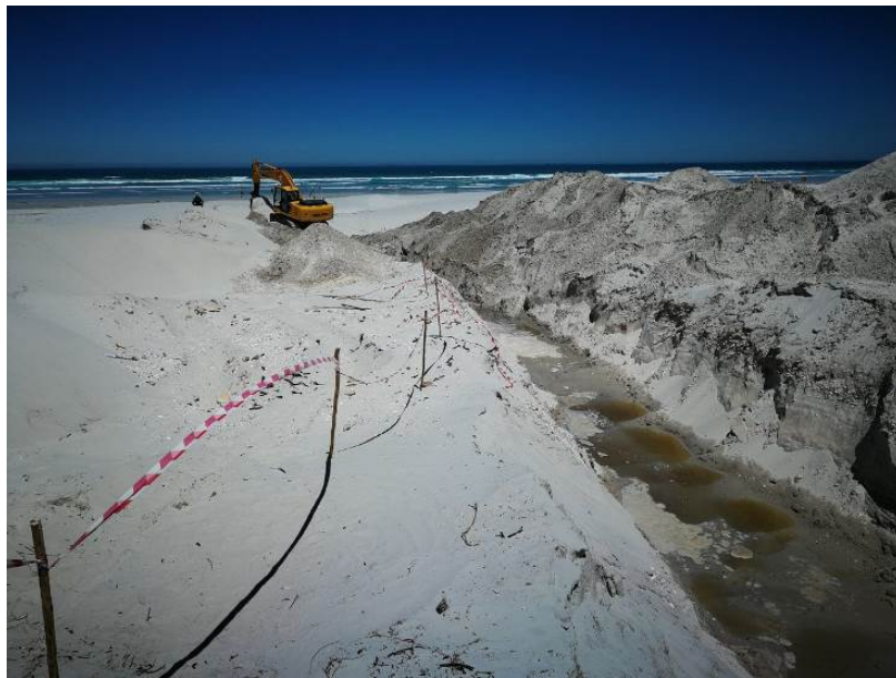
Figure 8 Example of excavations to take place on Melkbosstrand Beach to bury the submarine cable
