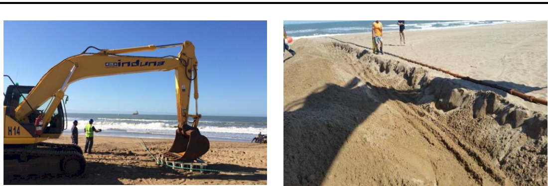
Plate 6 Landing of the cable on shore. Similar works will be undertaken for the landing of the Equiano Cable System
