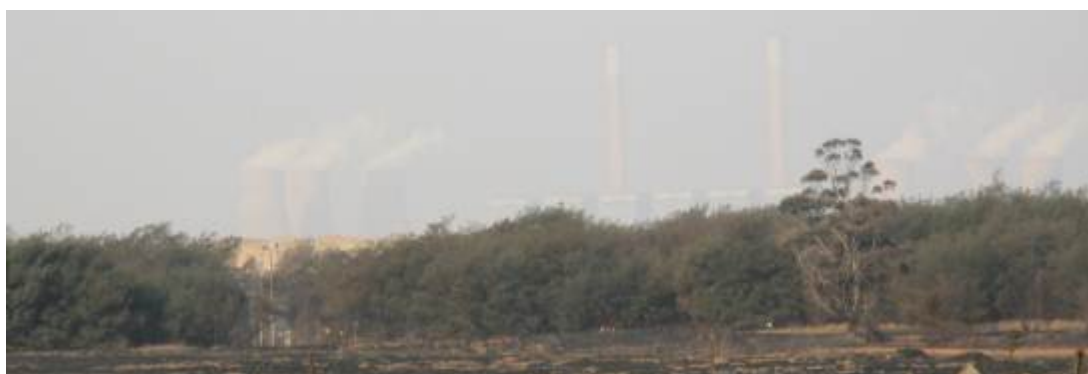
Figure 7-12: Photograph of Duhva power station
