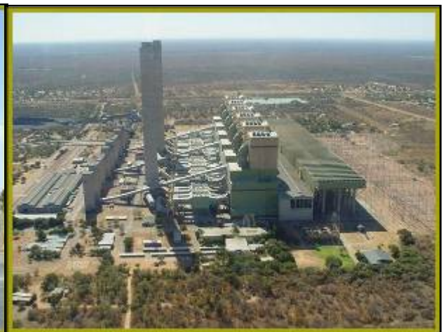
Figure 3-9: Photograph showing a power station with direct dry cooling technology
