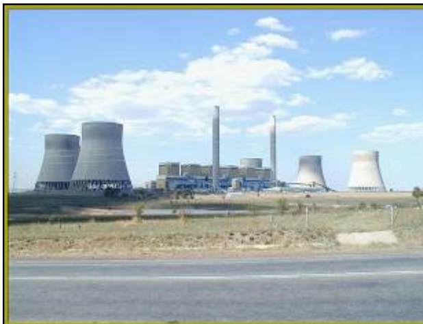
Figure 3-8: Photograph showing a power station with indirect dry cooling technology
