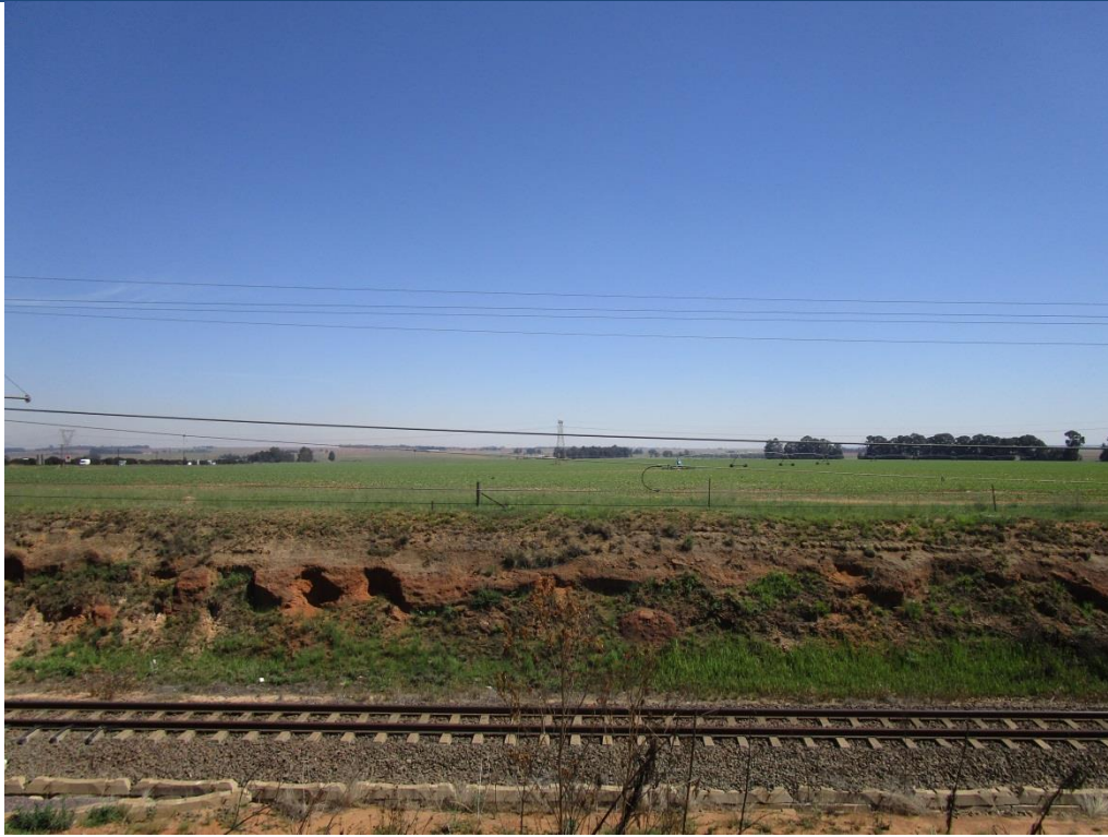
Photo 5: A view of the existing Bothashoek/Speculate power line in the distance.
