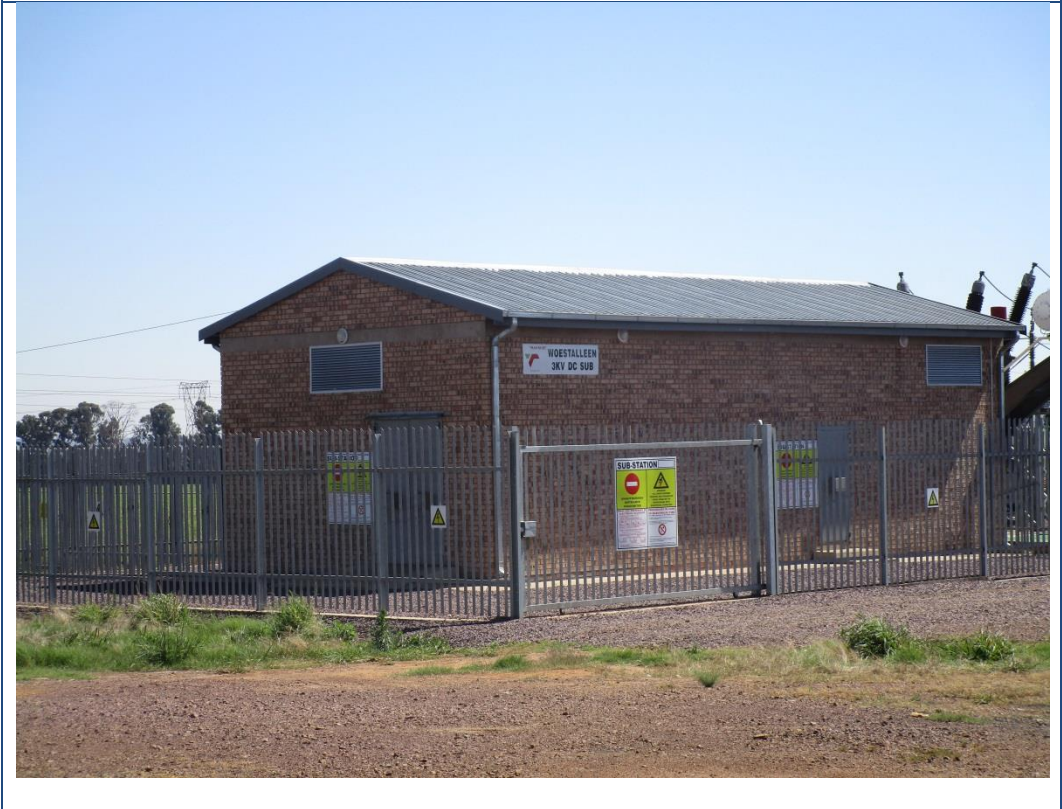
Photo 4: The existing Transnet Woestalleen traction substation
