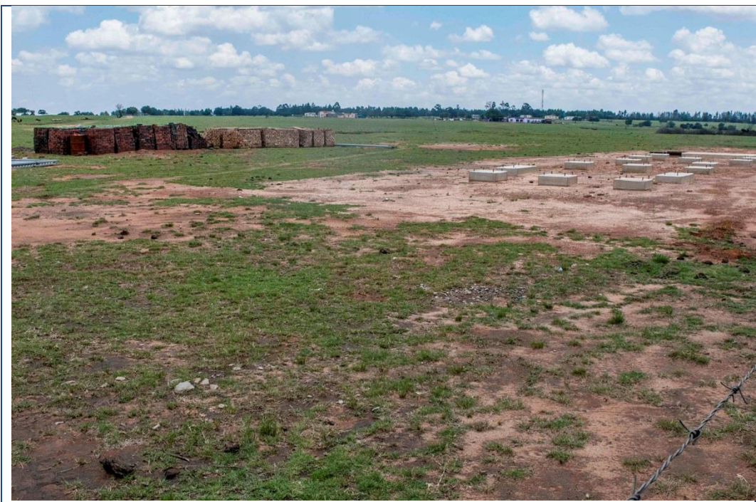
Photo 3: The new substation under construction.
