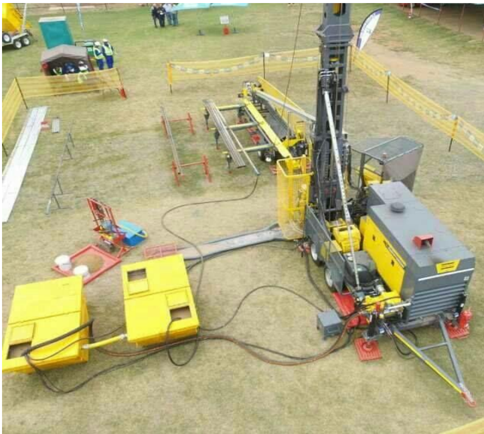
Figure 7: Typical examples of drill rig site
