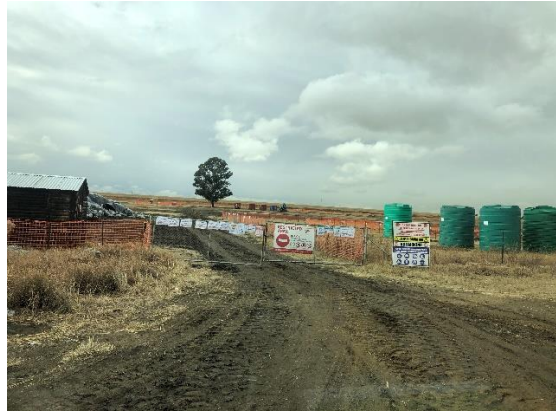
8.Soil remediation on project area
