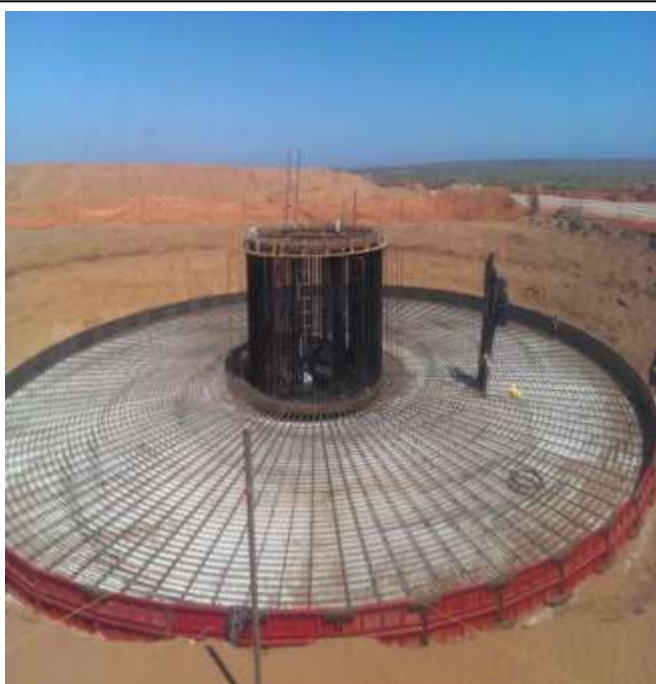
Figure 7.1: Concrete foundation (Eskom Sere Wind Facility)
